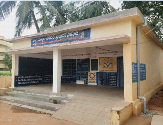
Photograph of the pre-primary school after fixing the PVC pipe to the roof
