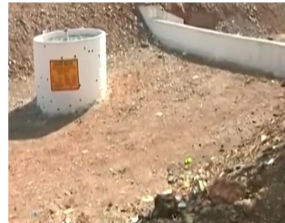
Construction of Water Conservation Pit in an Innovative Manner
