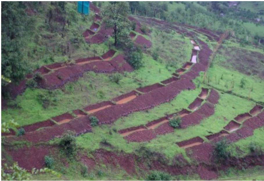
Method of Storing Rainwater in a Hilly Area by Contouring Method
