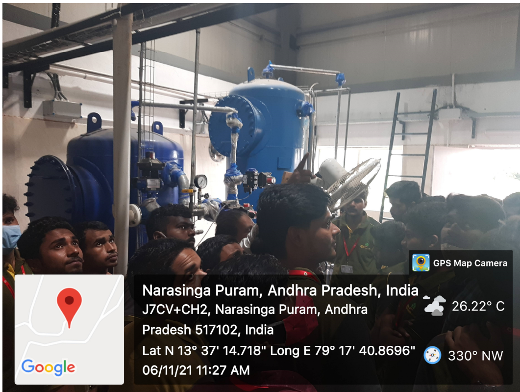
Students observing Water Treatment Plant in Smart Kitchen Building, SVEC
