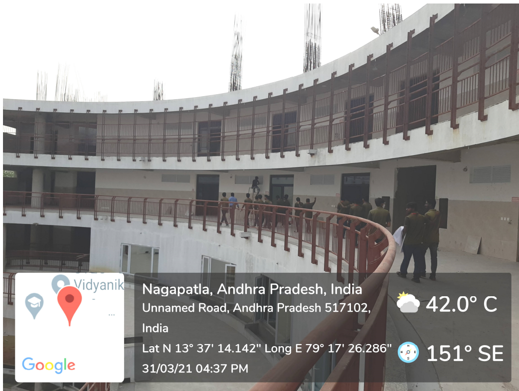
Photographs at Construction Site of New Academic Block G+8 Floors, SVEC Campus
