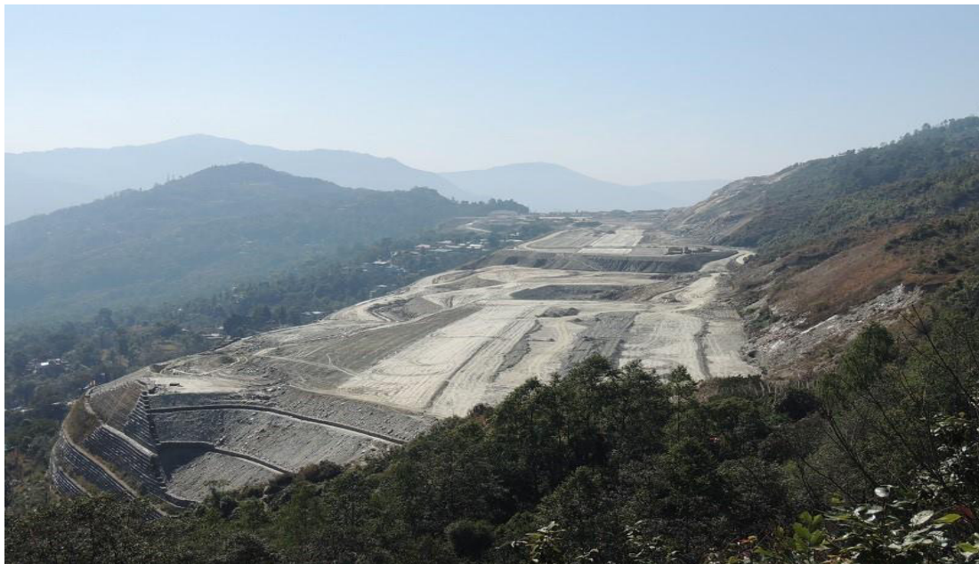
Photograph of Pakyong Airport Under Construction View as Part of Presentation
