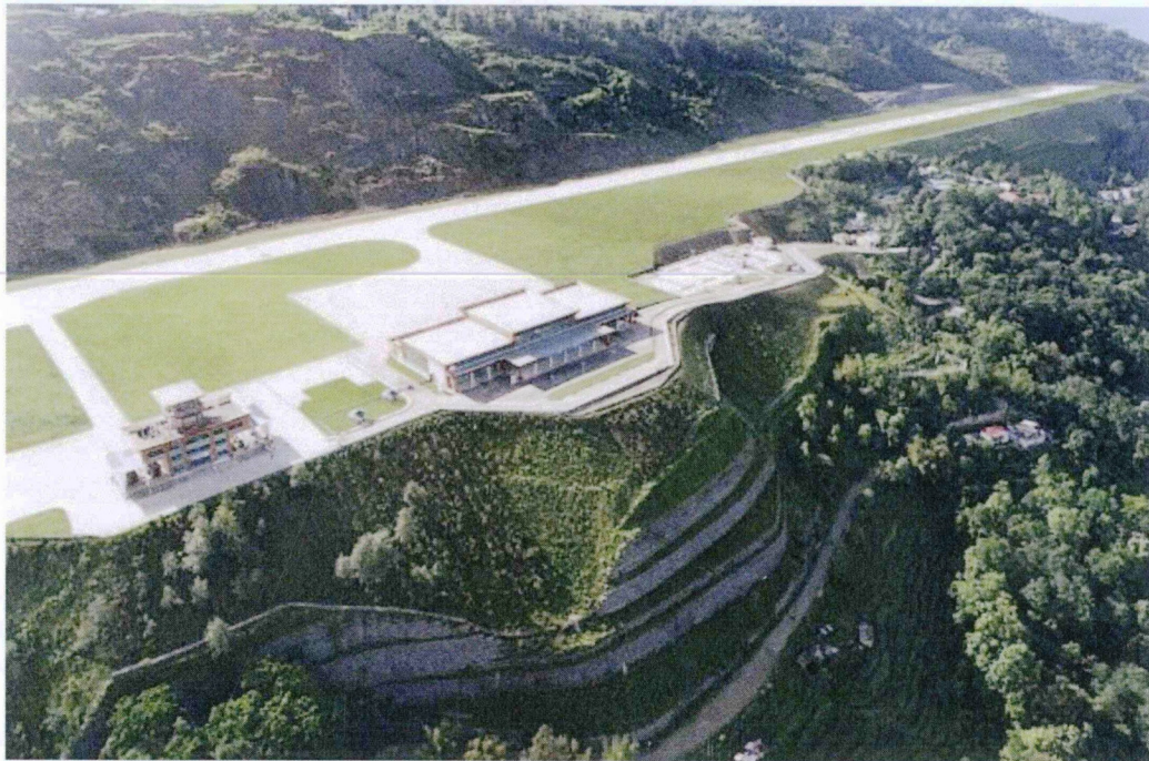
Photograph of Pakyong Airport After Construction View as Part of Presentation
