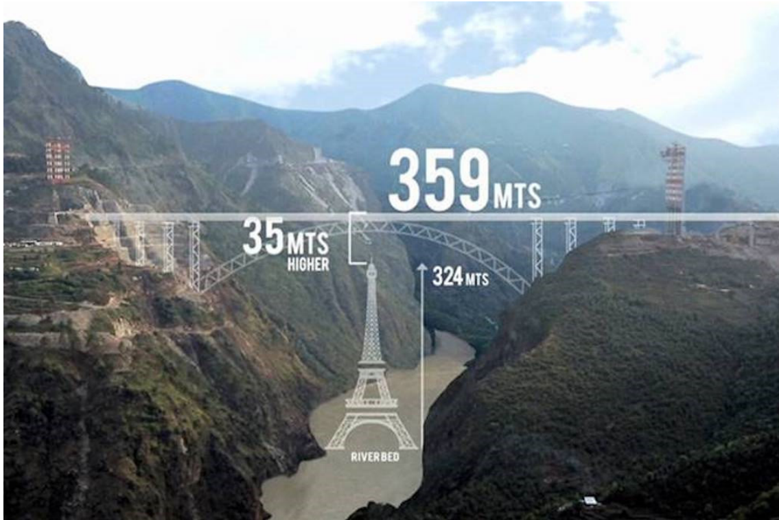
Photograph of World's Highest Railway Bridge - Chenab Railway Bridge Construction as part of presentation
