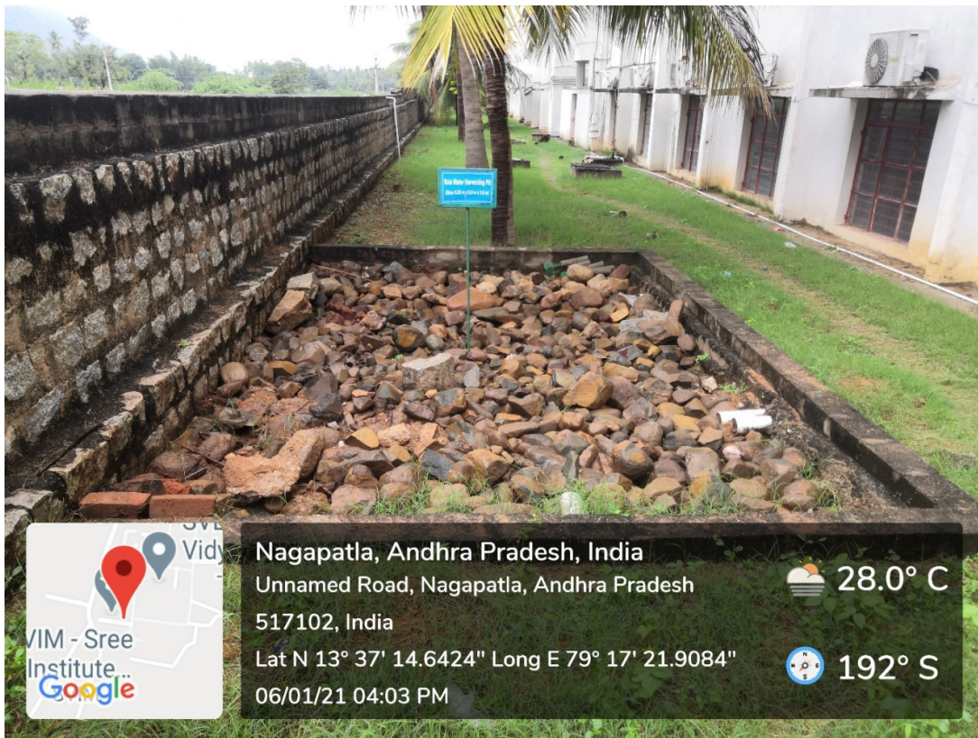
Rainwater Harvesting Pit beside MNS Block (Size: 5.25 m x 5.0 m x 3.6 m)
