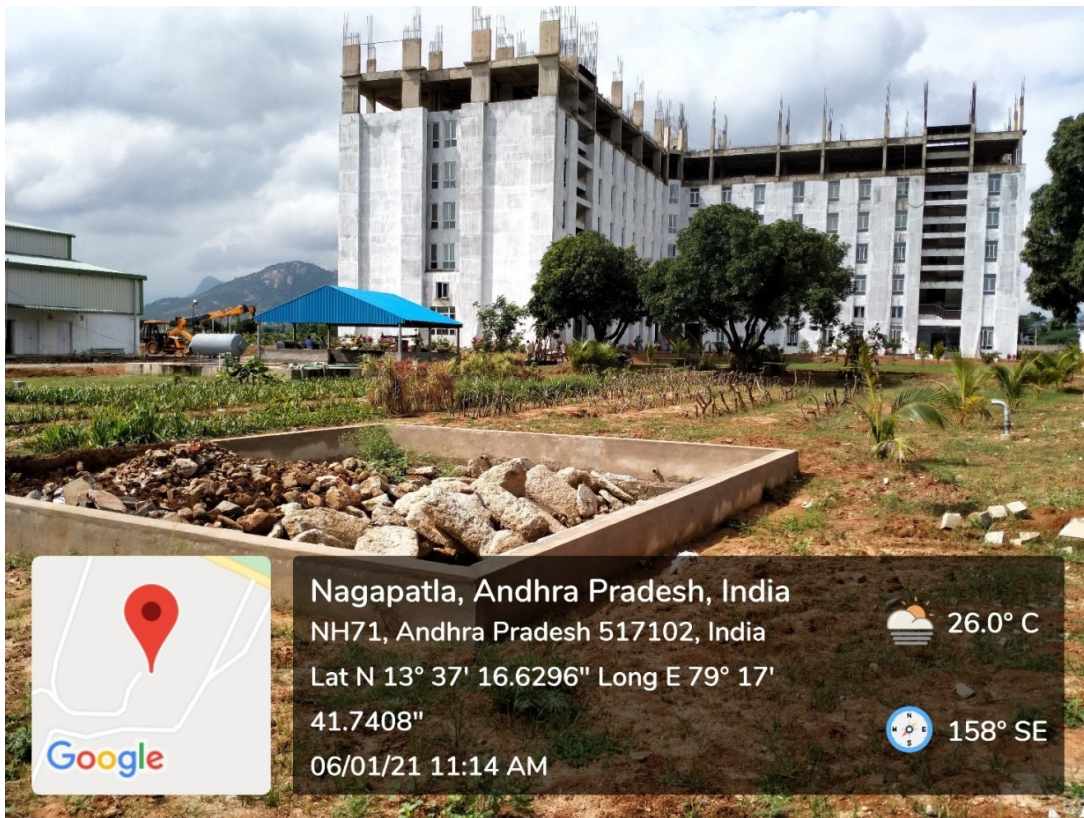
Rainwater Harvesting Pit at East of V Block (Size: 8.8 m x 7.8 m x 3.6 m)
