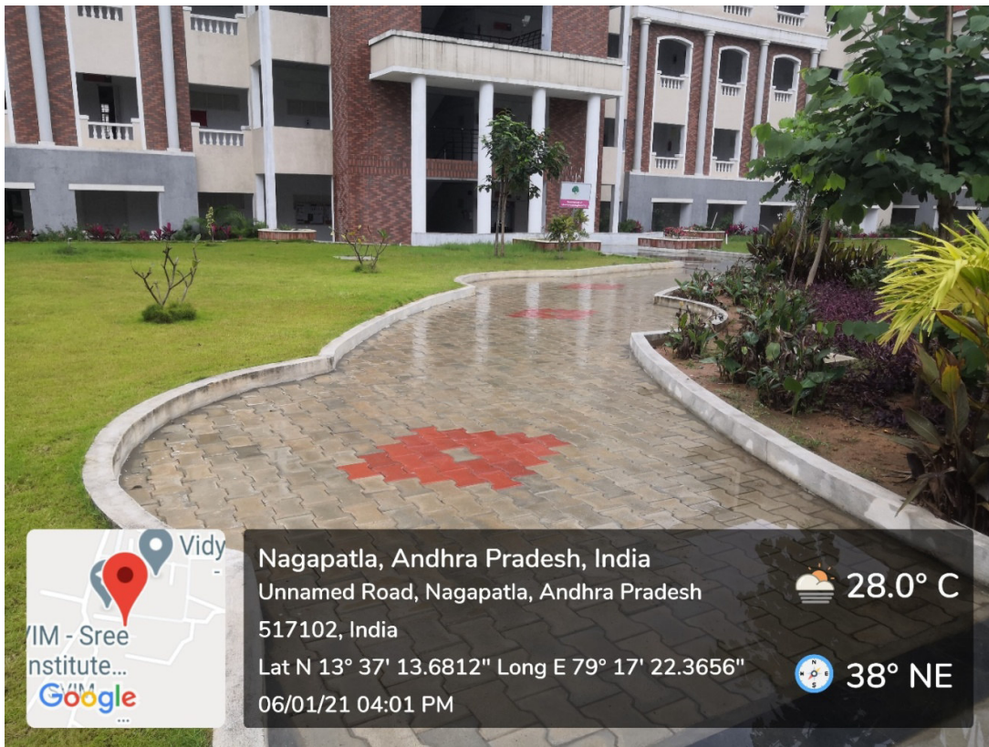
Porous/Permeable Concrete Paver Tiles Separated by Joints in Front of Mechanical Engineering Block to Infiltrate Rainwater
