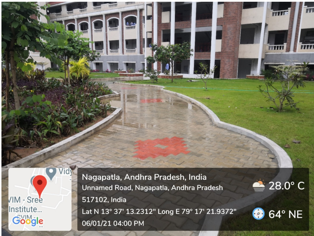
Porous/Permeable Concrete Paver Tiles Separated by Joints in Front of Civil Engineering Block to Infiltrate Rainwater
