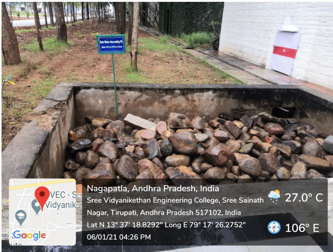
Rainwater Harvesting Pit at PAT Office (Size: 4.0 m x 4.0 m x 3.6 m)
