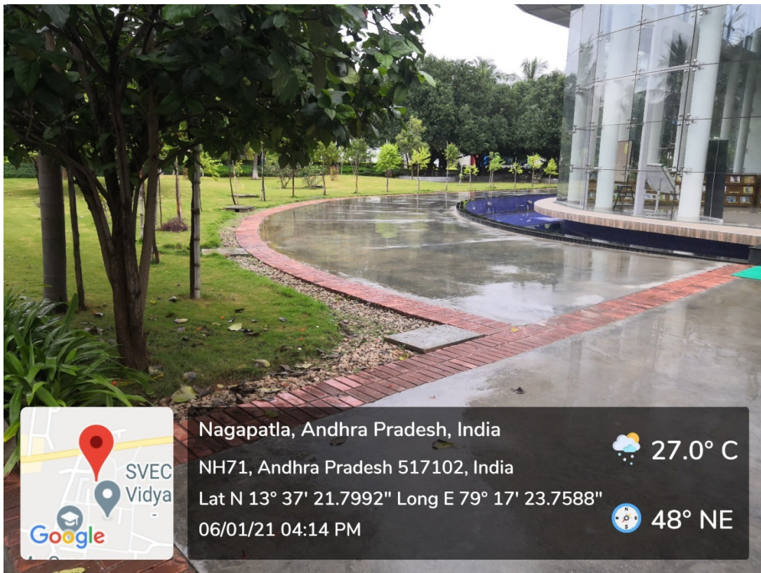
Rain Water Collection Point at Central Library
