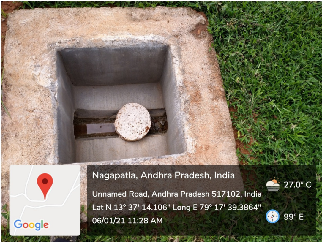
Rain Water Collection Point at V Block
