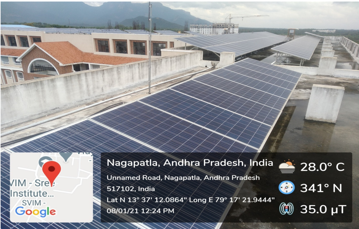
Roof Top Solar Power Plant at Civil Engineering Block South
