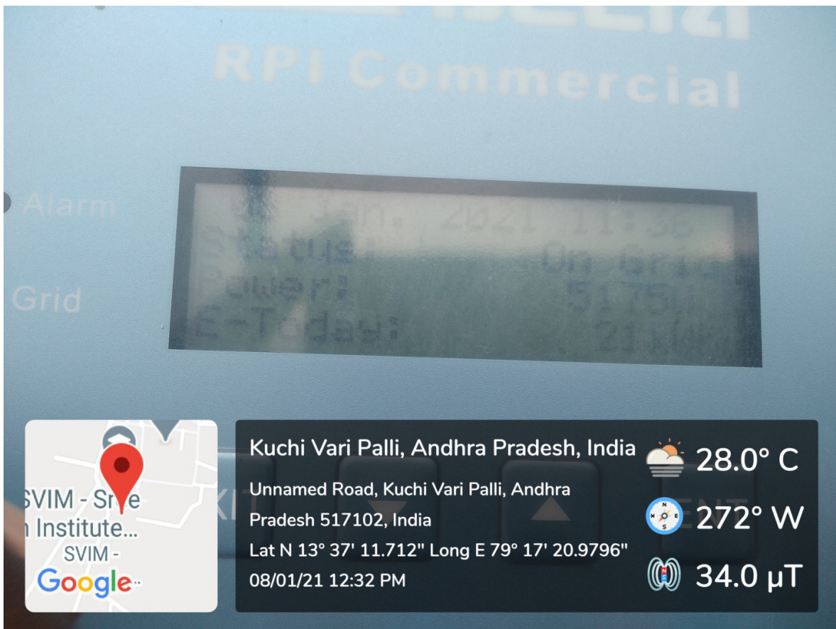
Indication of Roof Top Solar Plant Grid Connection
