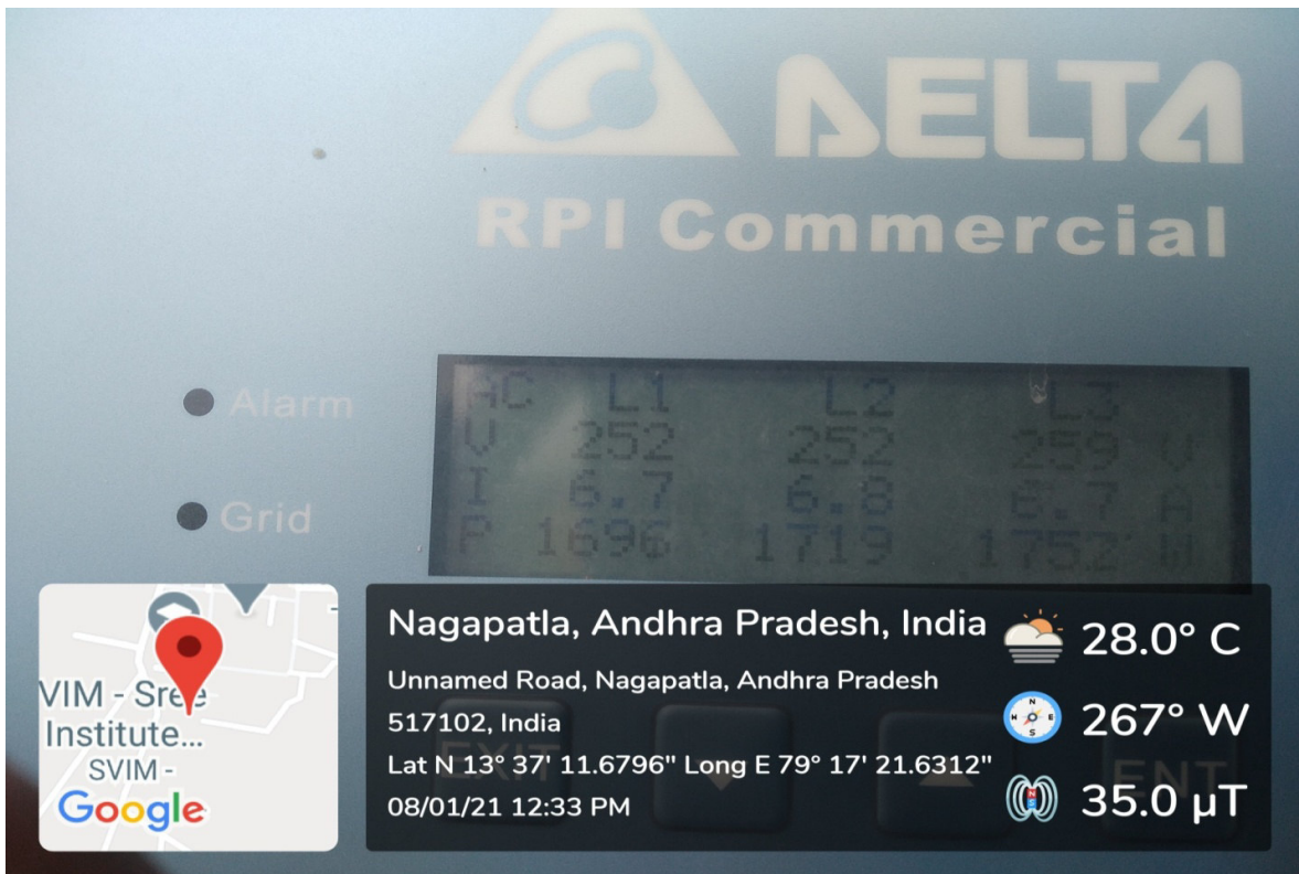
Roof Top Solar Plant Grid Three Phase Supply Levels
