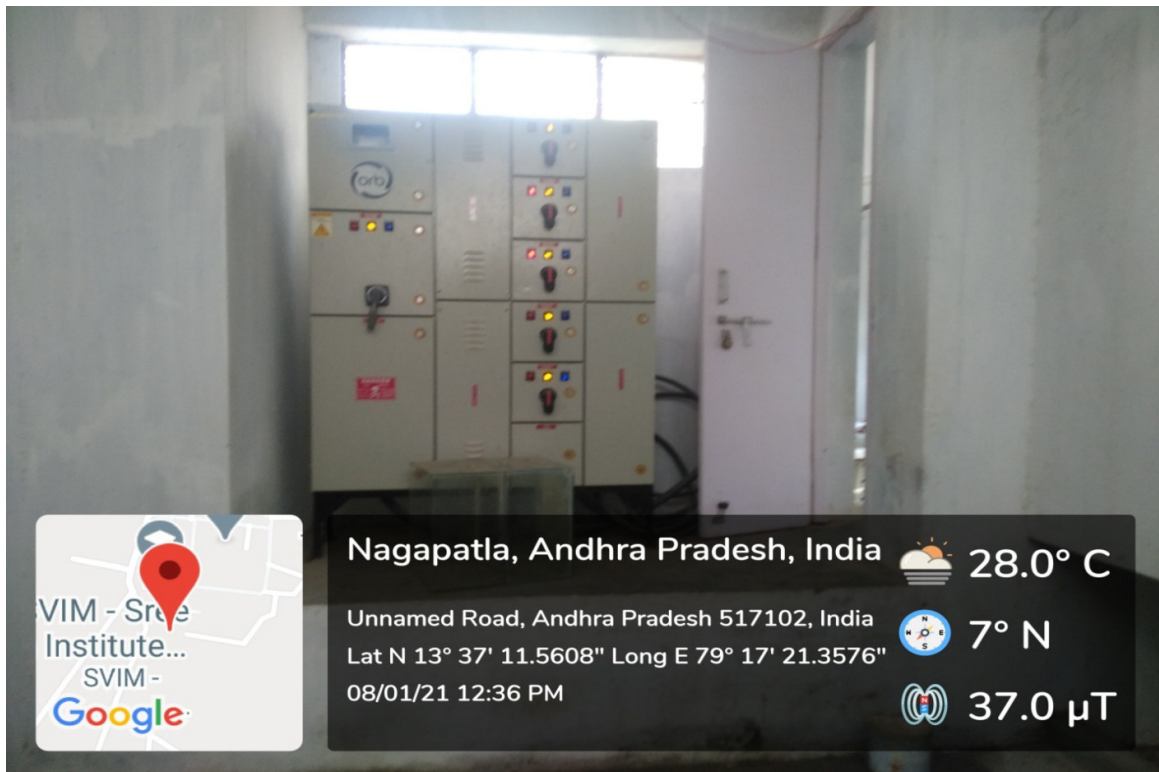
Inverter Switch Gear Panel for connecting Roof Top Solar Plant to Grid
