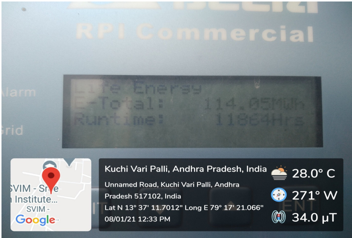
Roof Top Solar Plant Grid Connection Measurements
