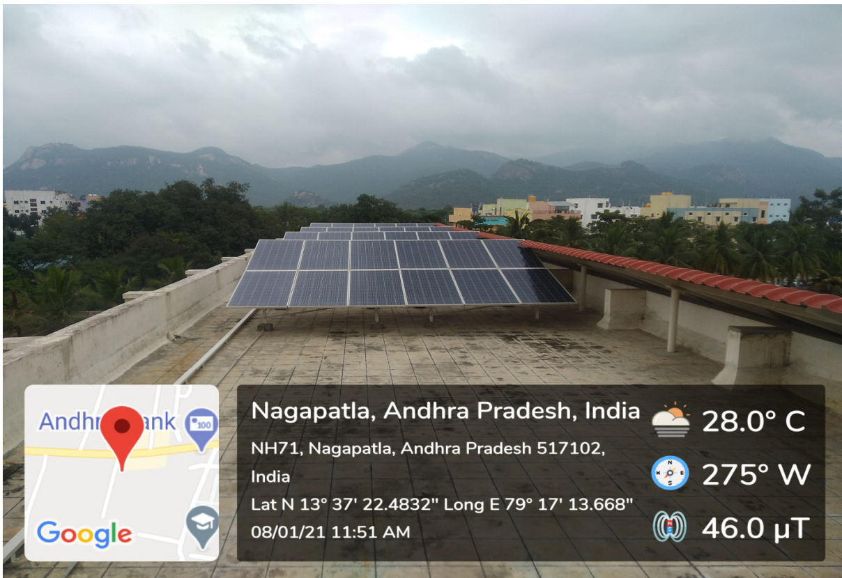
Roof Top Solar Power Plant at PG Block
