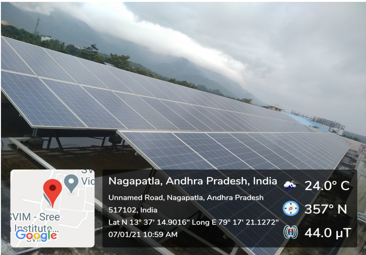
Roof top Solar Power Plant at MNS Block West
