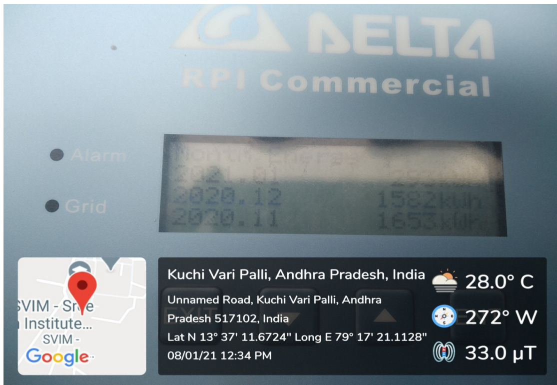
Roof Top Solar Plant Grid Connection Measurements (Month Wise Indication)
