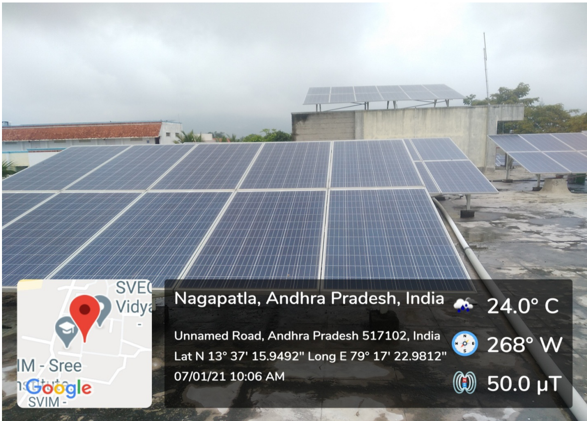
Roof Top Solar Power Plant at West Wing of M-Plaza
