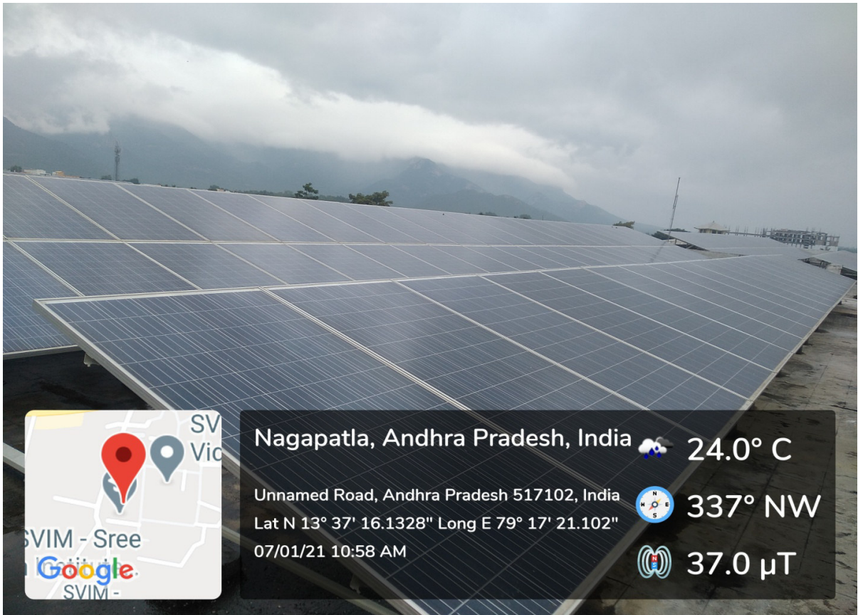
Roof top Solar Power Plant at MNS Block North
