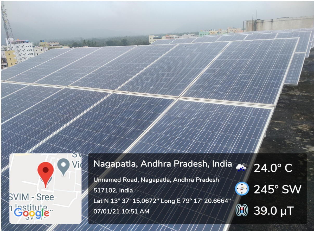
Roof Top Solar Power Plant at MNS Block South
