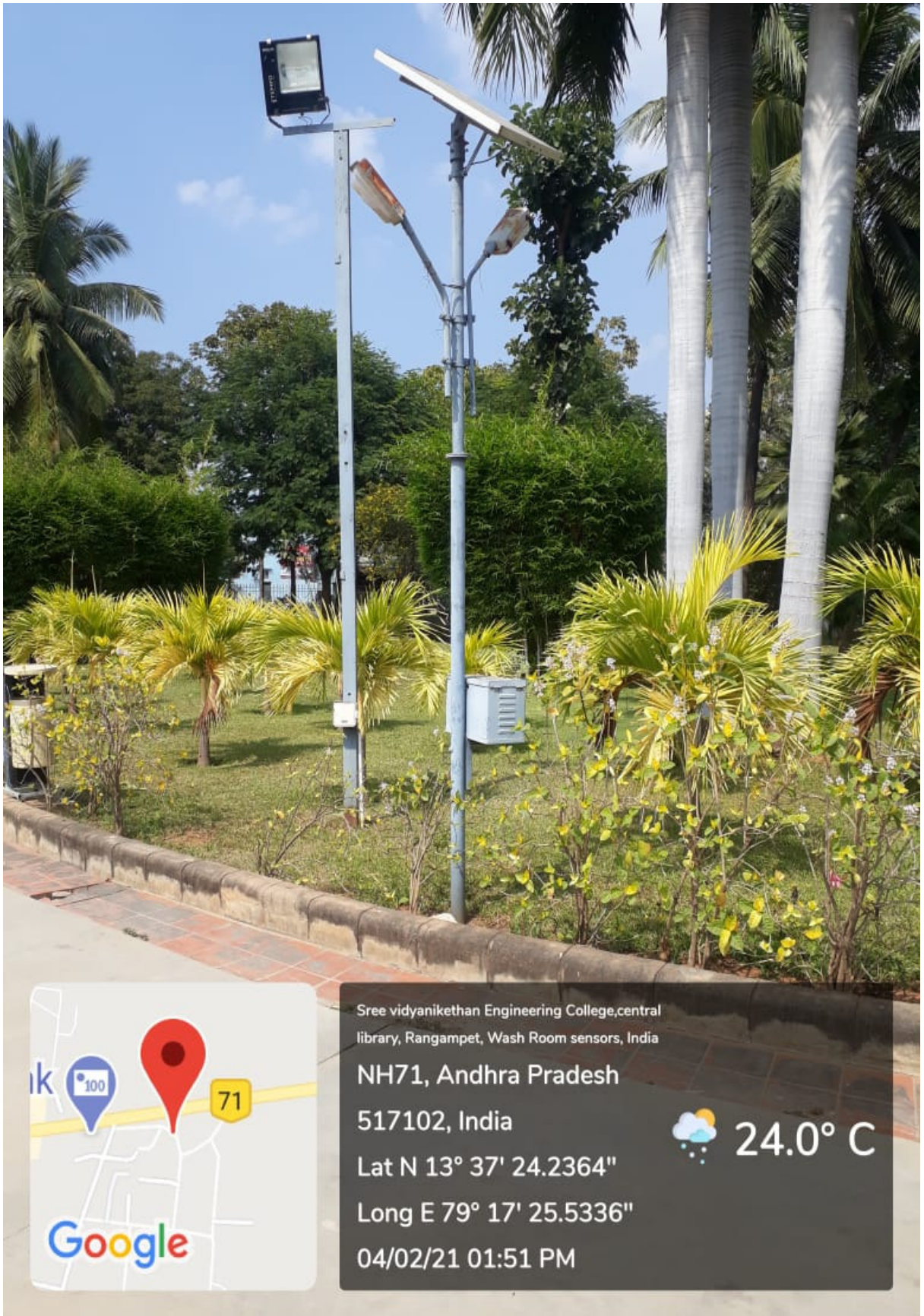
Solar Street Light at the Entrance of the College
