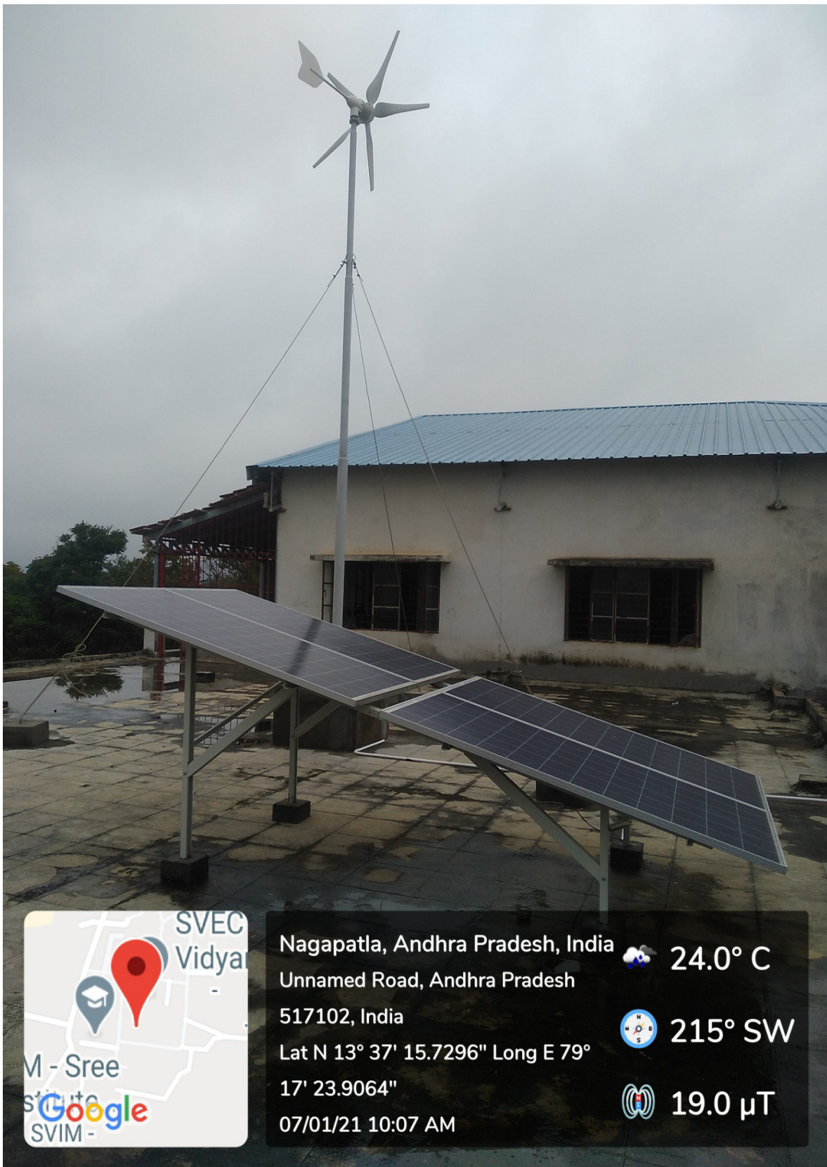
1.6 kWp WISH SYSETM (Roof Top Solar and Wind Integrated System) at Centre for Energy Research Lab
