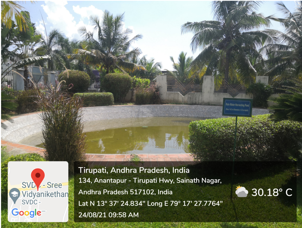
Rain Water Harvesting Pond at Main Gate (Size: 14.5 m Diameter X 1.5 m Depth)
