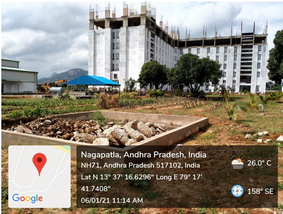
Rainwater Harvesting Pit at East of V Block (Size: 8.8 m x 7.8 m x 3.6 m)
