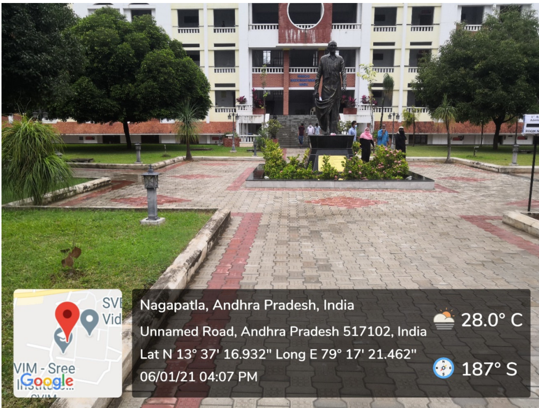
Porous/Permeable Concrete Paver Tiles Separated by Joints at MNS Block to Infiltrate Rainwater
