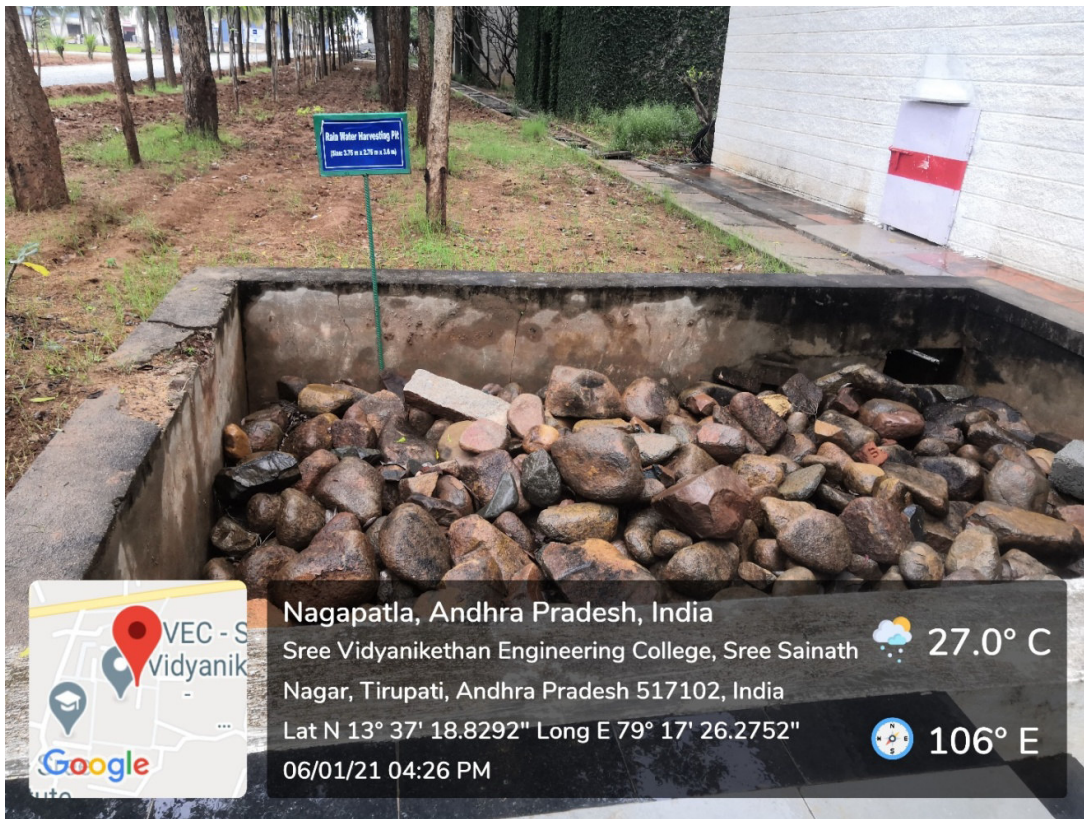
Rainwater Harvesting Pit at PAT Office (Size: 4.0 m x 4.0 m x 3.6 m)
