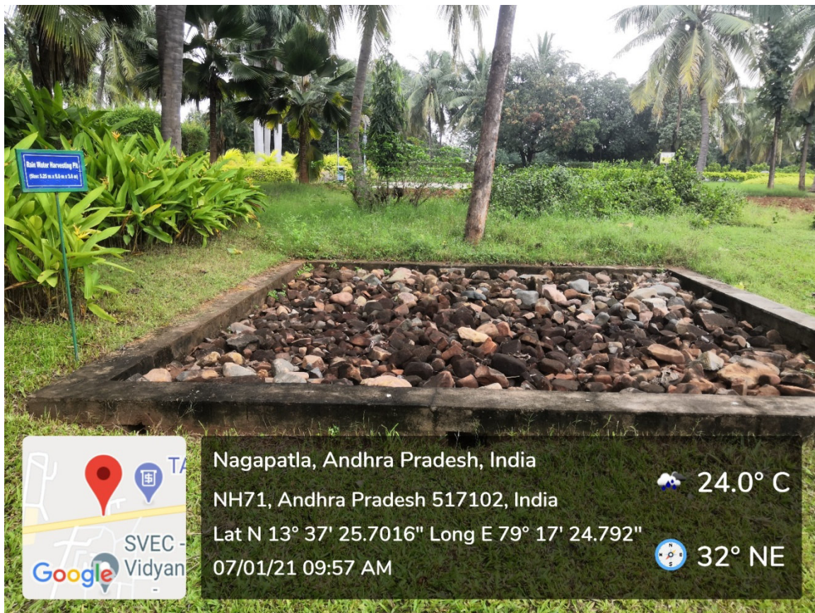
Rainwater Harvesting Pit at New Canteen (Size: 5.25 m x 5.0 m x 3.6 m)
