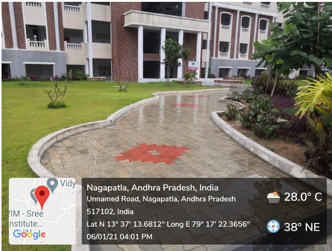
Porous/Permeable Concrete Paver Tiles Separated by Joints in Front of Mechanical Engineering Block to Infiltrate Rainwater
