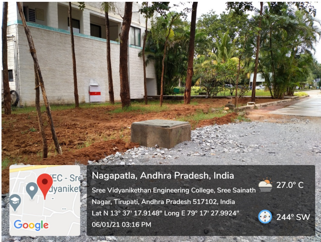
Rain Water Collection and Conveyance System at PAT Office
