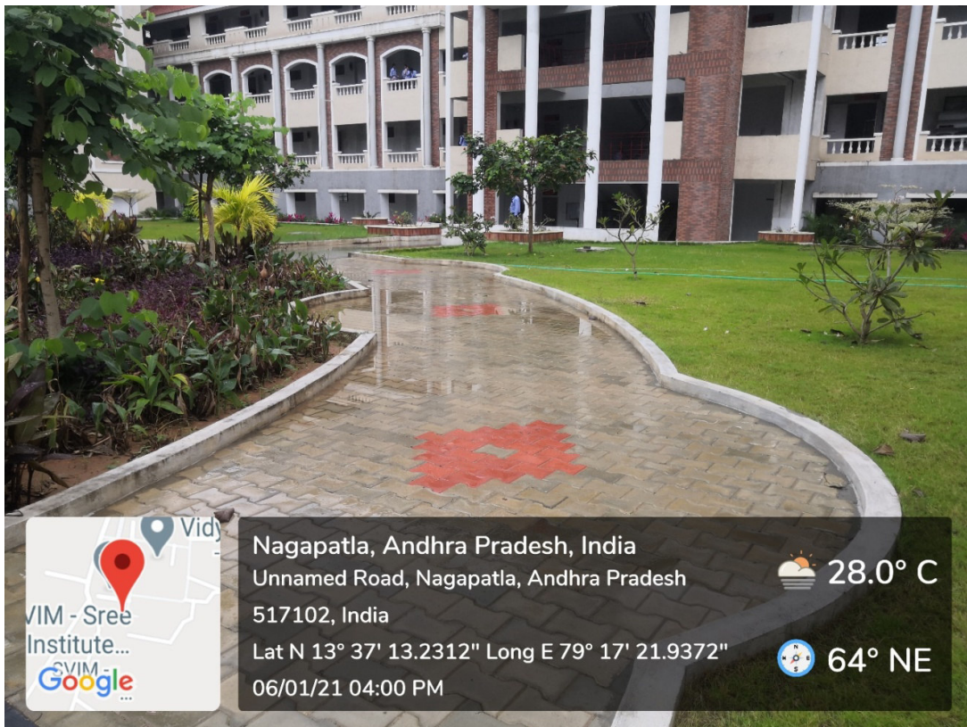
Porous/Permeable Concrete Paver Tiles Separated by Joints in Front of Civil Engineering Block to Infiltrate Rainwater
