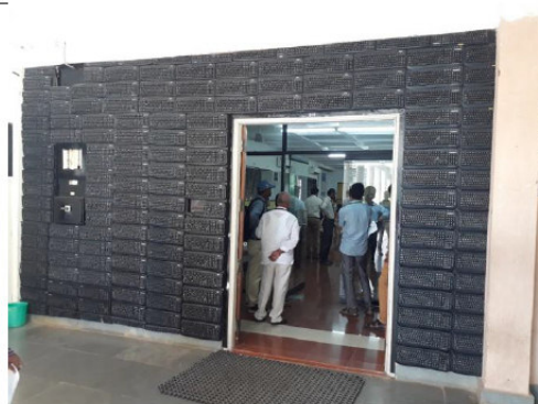
Reuse of discarded electronic items on the wall (Key Boards)
