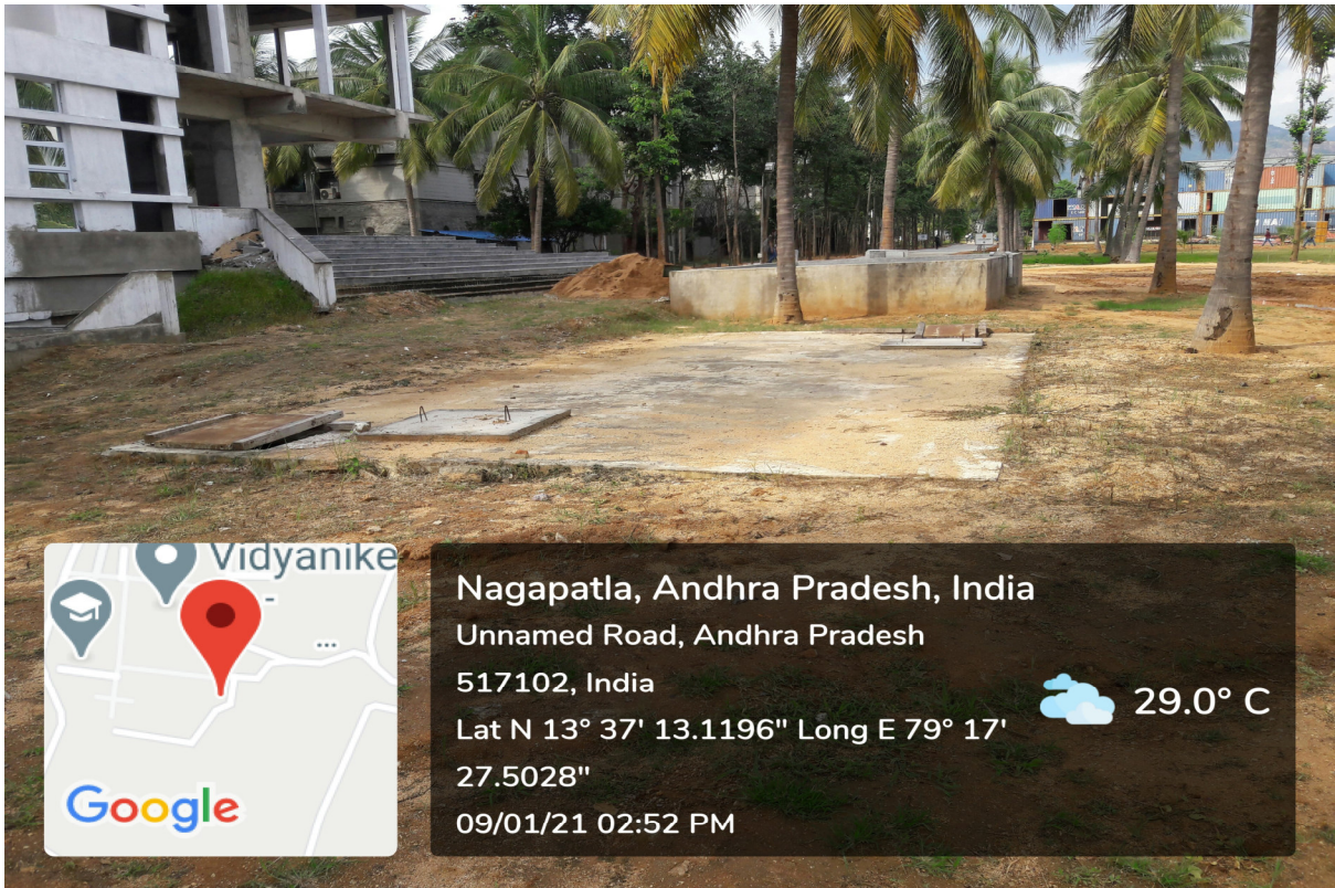
Underground Tank at Academic Block of Size: 9.3 m x 5.4 m x 3 m and Capacity: 150000 Litres
