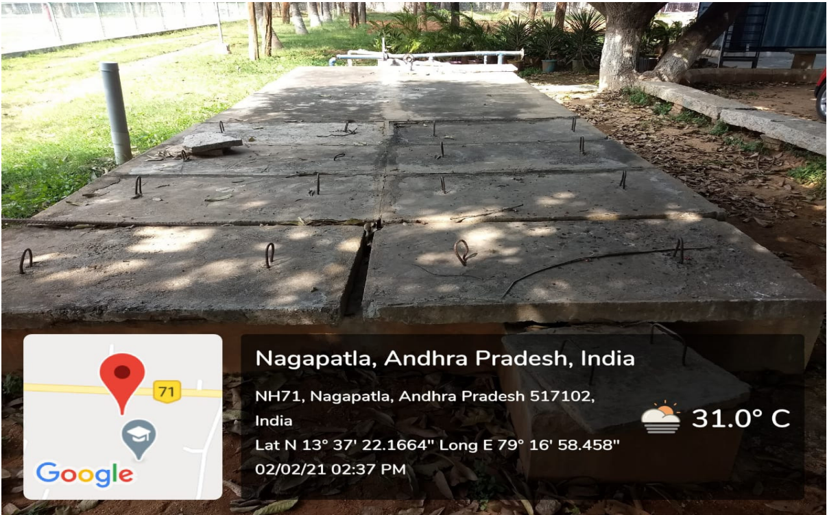
Underground Tank at Girls Hostels of Size: 8.8 m x 3.2 m x 3.6 m and Capacity: 101,000 Litres
