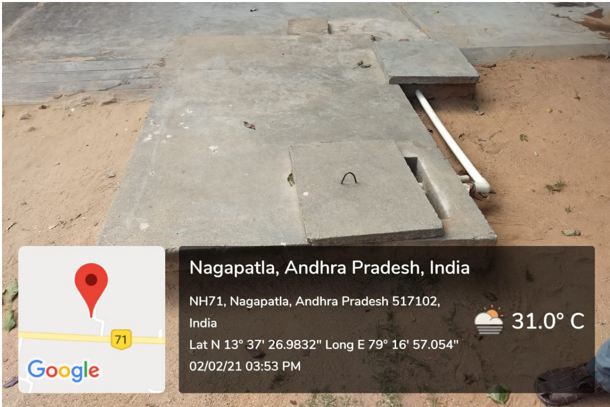
Underground Tank at SS1 Block, Boys Hostels of Size: 2.4 m x 1.5 m x 3 m and Capacity: 10000 Litres
