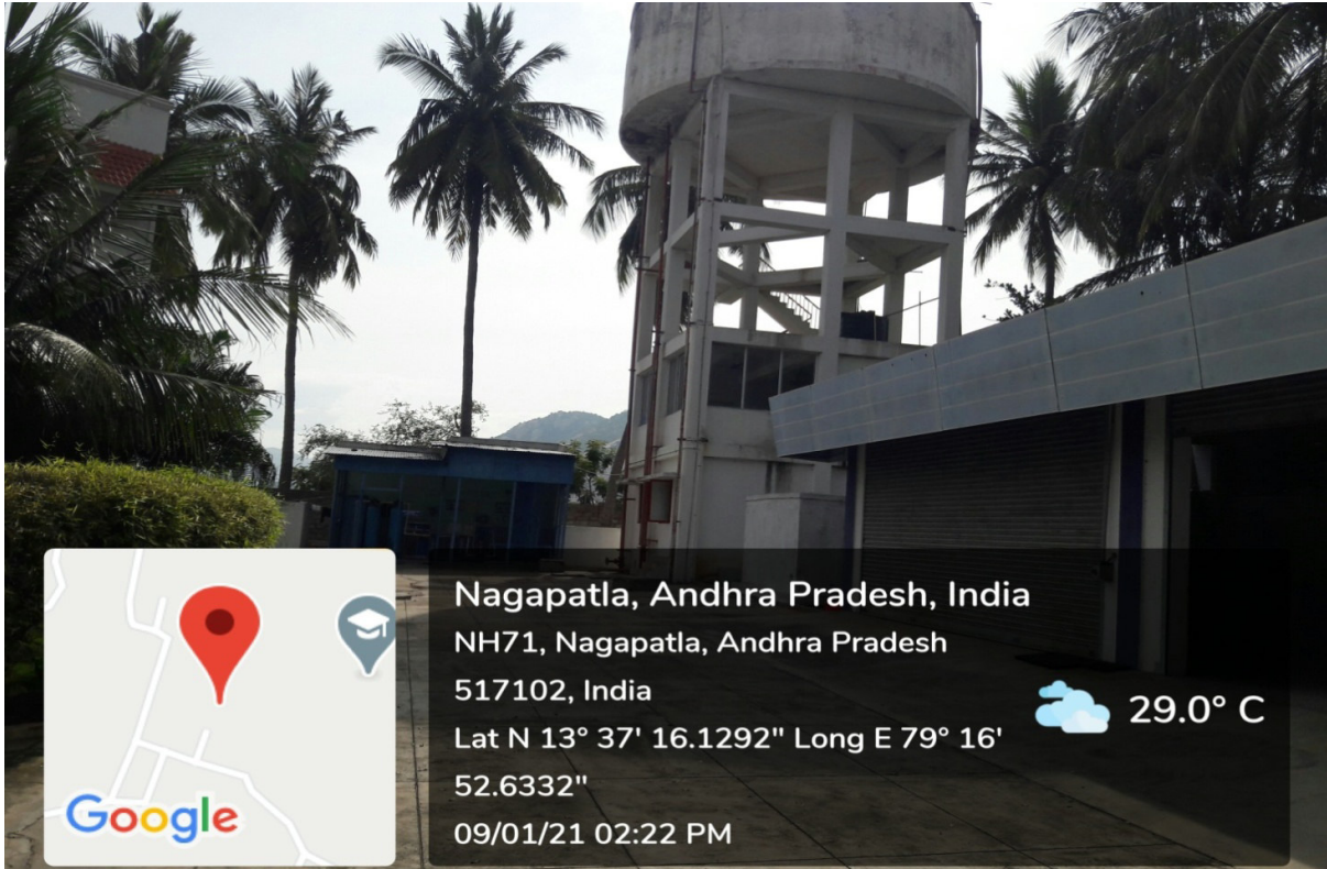
Overhead Tank at Girls Hostels of Size: 9.3 m Diameter x 4 m Height and Capacity: 271000 Litres
