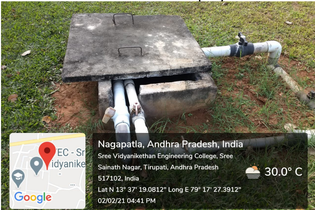
Underground Tank at PAT Office of Size: 7 m x 4 m x 2.5 m and Capacity: 70, 000 Litres
