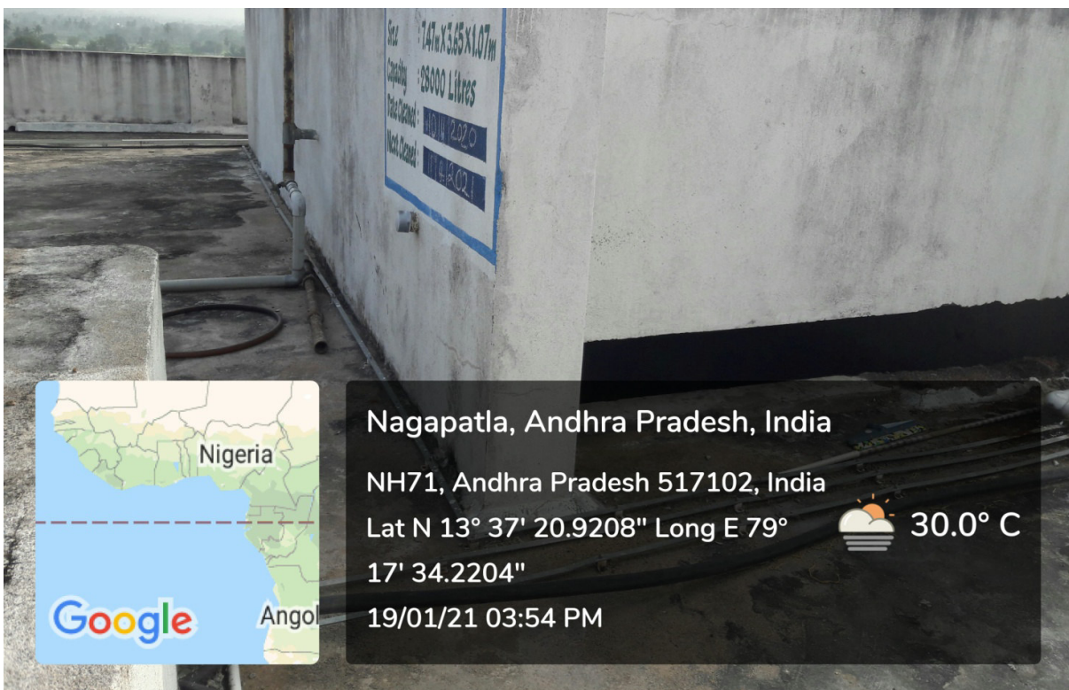
Overhead Tank (Terrace) at Civil Engineering Block South of Size: 7.47 m x 3.65 m x 1.07 m and Capacity: 28000 Litres
