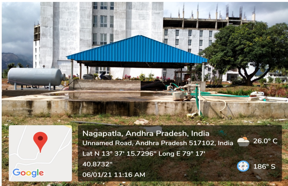
Underground Water Storage Tank at V Block of Size: 10 m x 9.5 m x 3 m and Capacity: 300000 Litres
