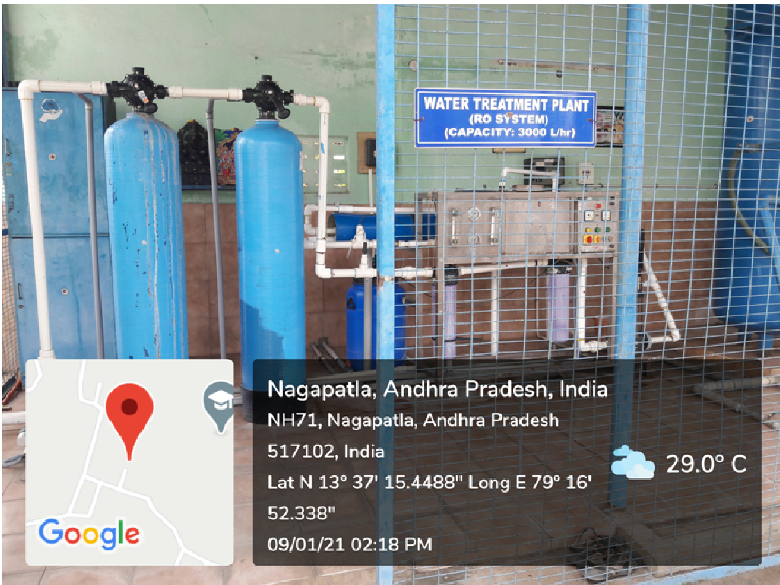
Reverse Osmosis (RO) System (3000 Liters per Hour Capacity) at Girls Hostel Premises
