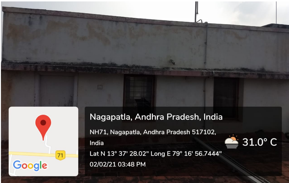
Overhead Tank at SS2 Block, Boys Hostels of Size: 8.3 m x 3.5 m x 1 m and Capacity: 29000 Litres
