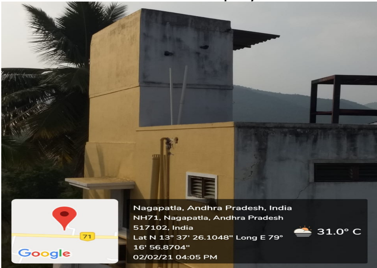
Overhead Tank at SS1 Block, Boys Hostels of Size: 3.5 m x 1.5 m x 1.6 m and Capacity: 8000 Litres
