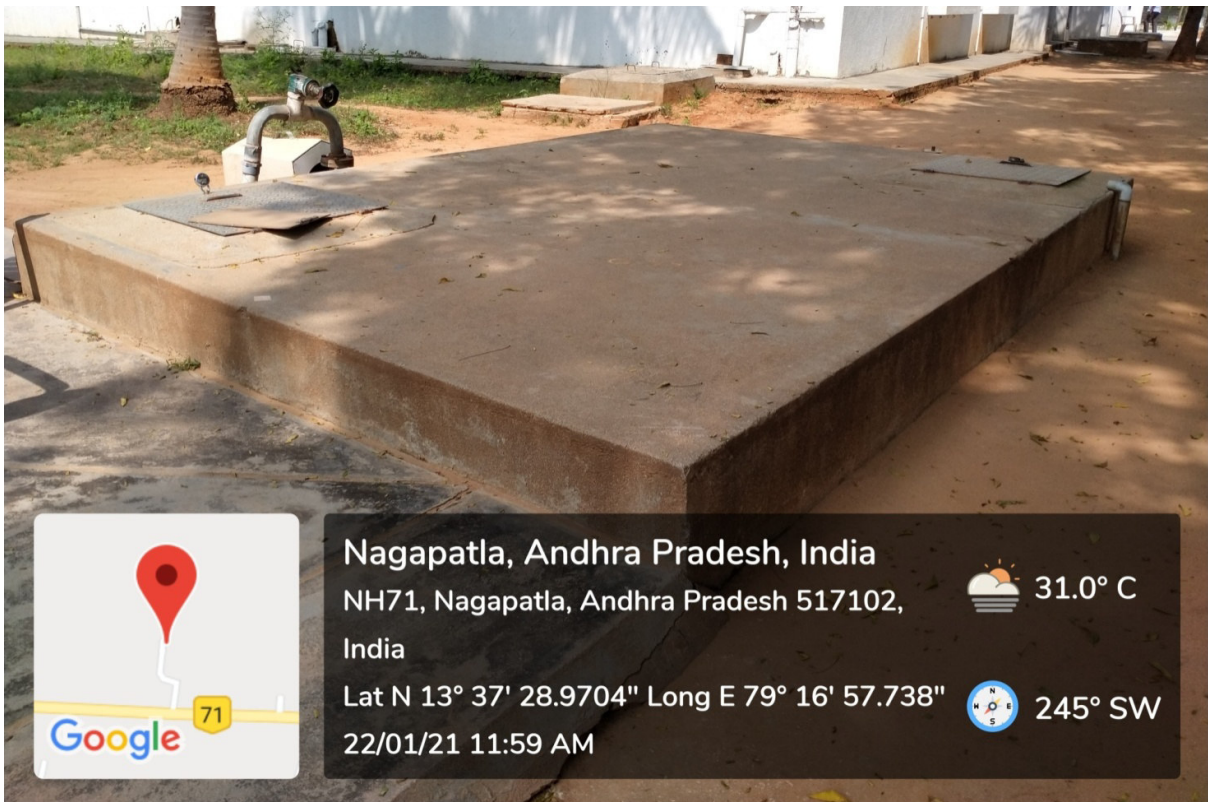
Underground Tank at SS2 Block, Boys Hostels of Size: 3.85 m x 2.71 m x 2.4 m and Capacity: 25000 Litres
