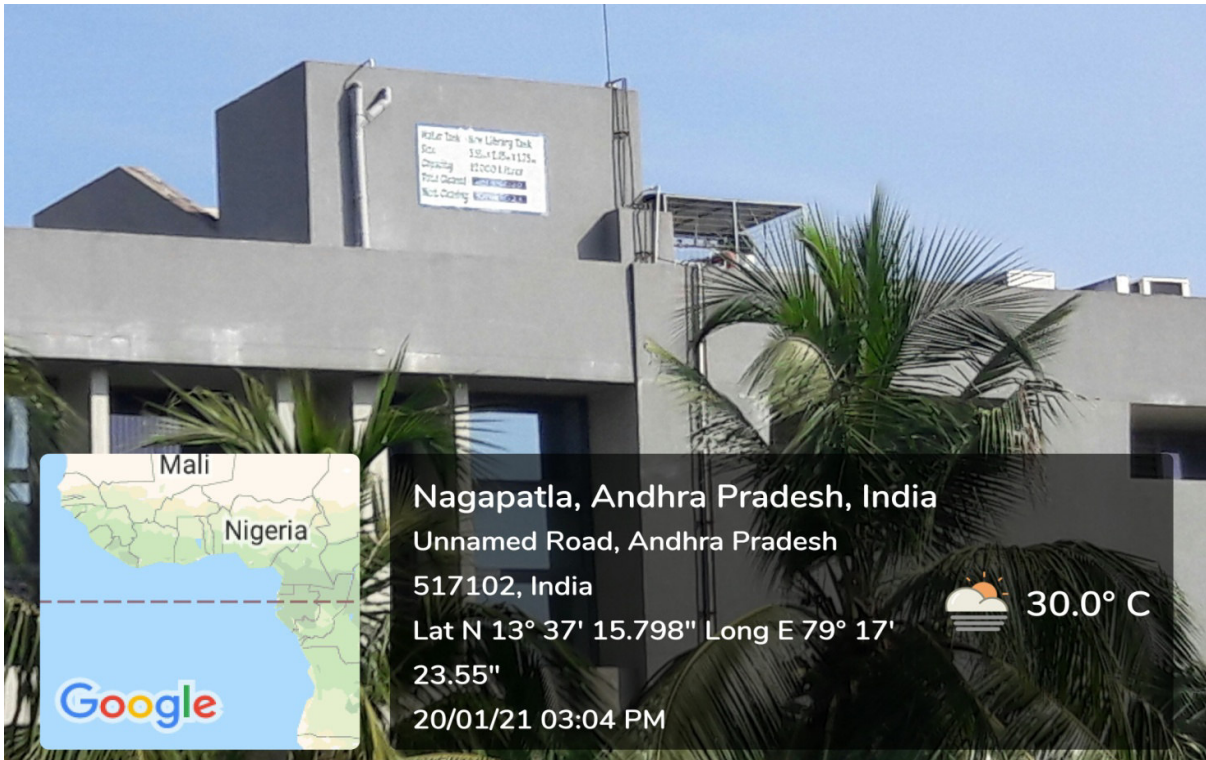
Overhead Tank at Central Library of Size: 3.35 m x 2.05 m x 1.75 m and Capacity: 12000 Litres
