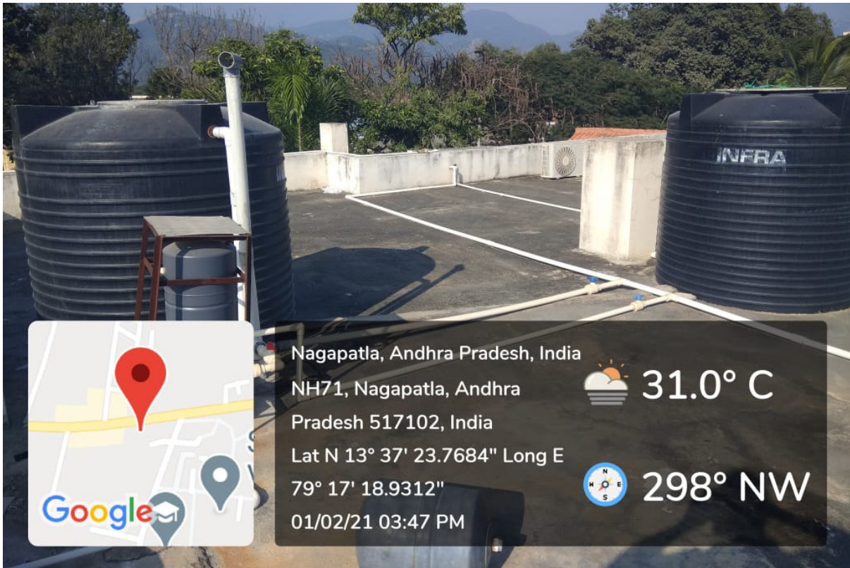
Overhead Tanks at Parents Guest House of 4000 Litres Capacity (2 Nos. - 2000 Litres Each)
