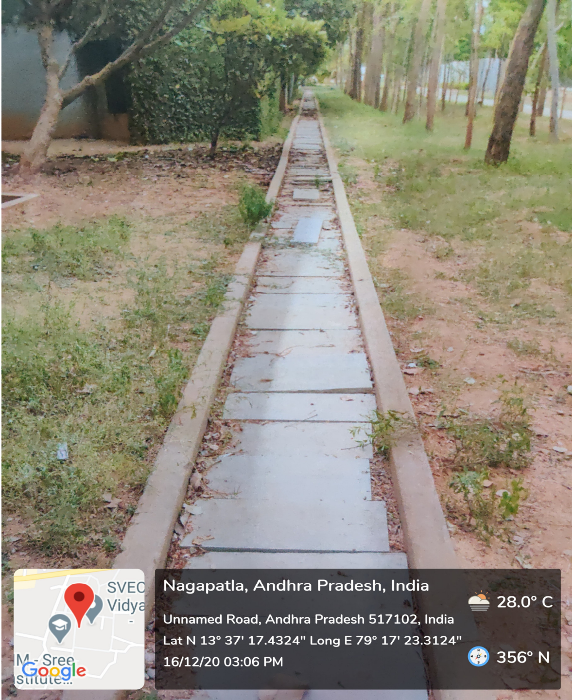
Underground Utility Duct for Cable Ways – A Sustainable Technology
