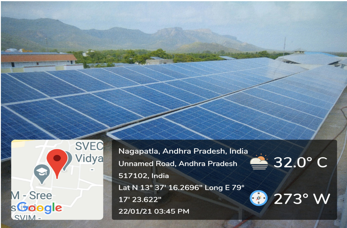
Roof Top Solar Power Plant of Capacity 500 KVA
