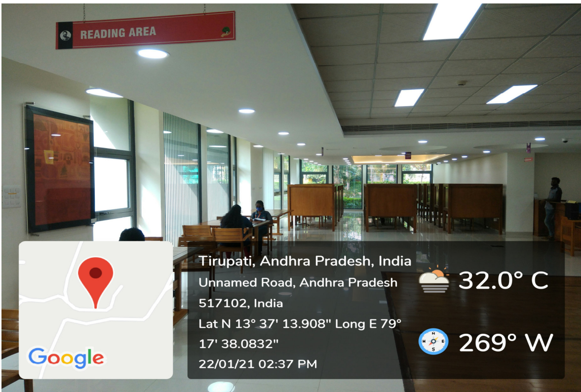
LED Lighting at Central Library
