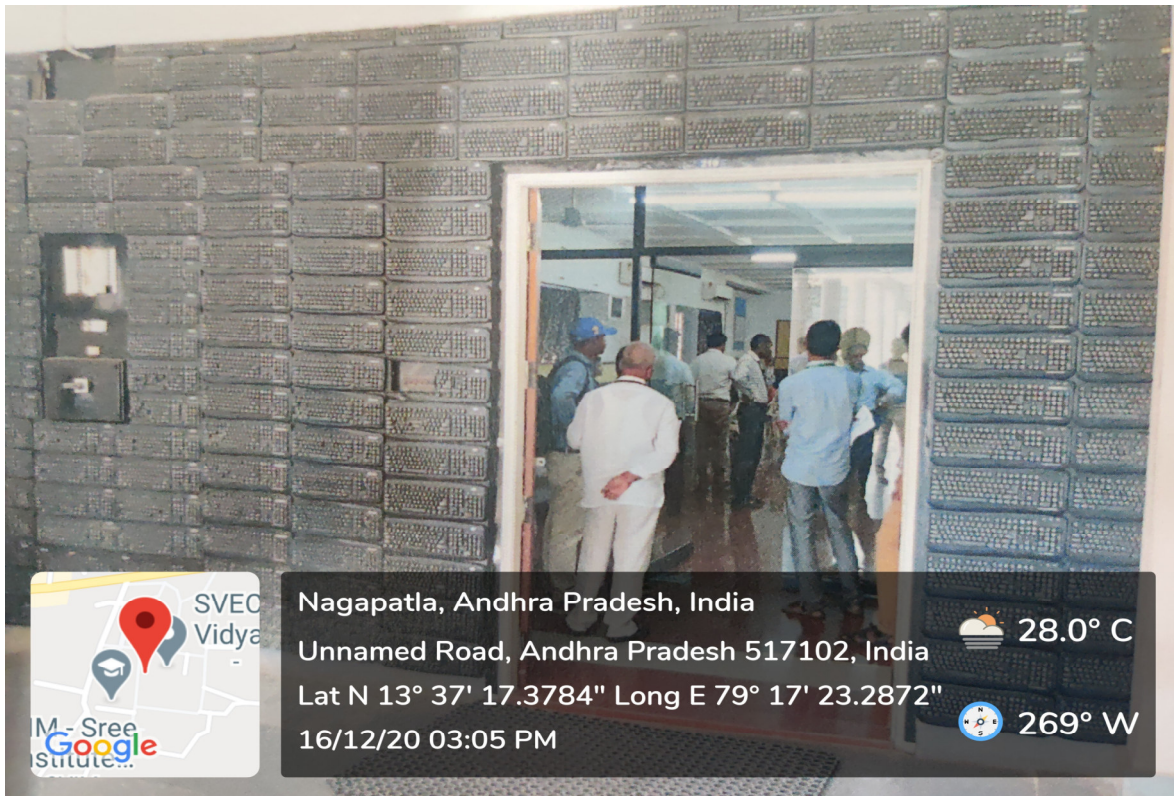
Computer Waste as Wall Cladding
