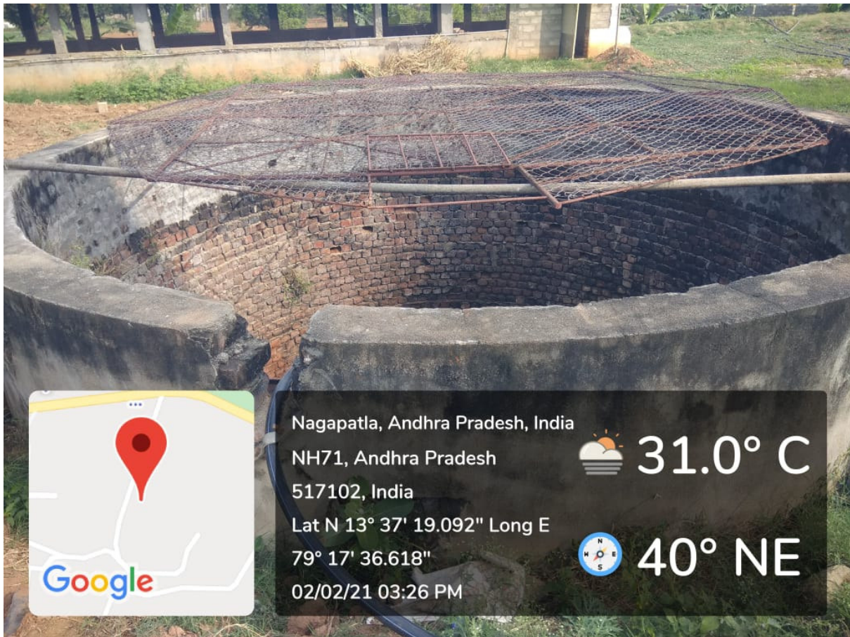
Open Well near V Block (Size: 5.13 m Diameter x 18 m Depth) with Bore (6.5" Diameter)
