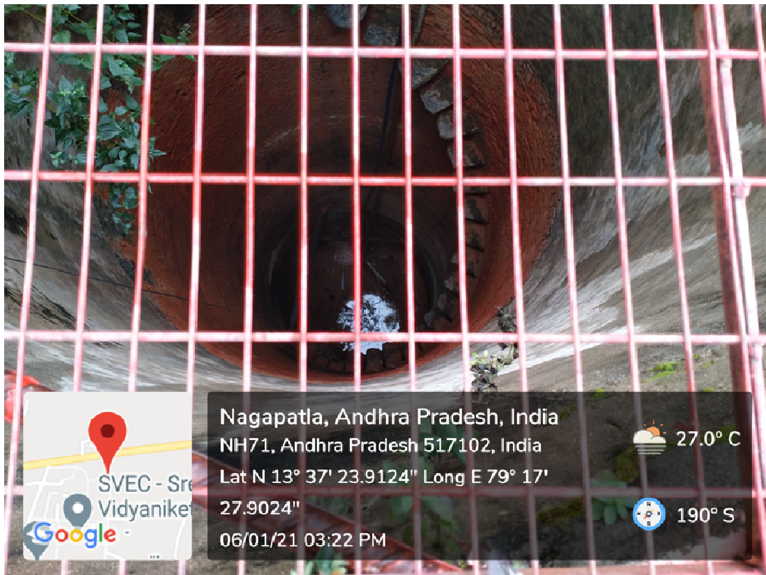
Open Well near Main Gate (Size: 4.3 m Diameter x 20 m Depth) with Bore (6.5" Diameter)
