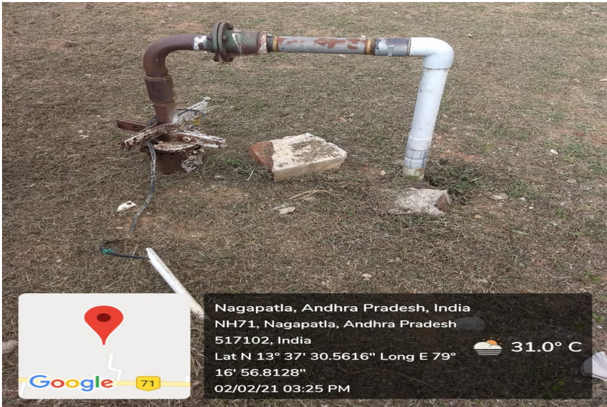
Bore Well-1 at Boys Hostel (8" Diameter)
