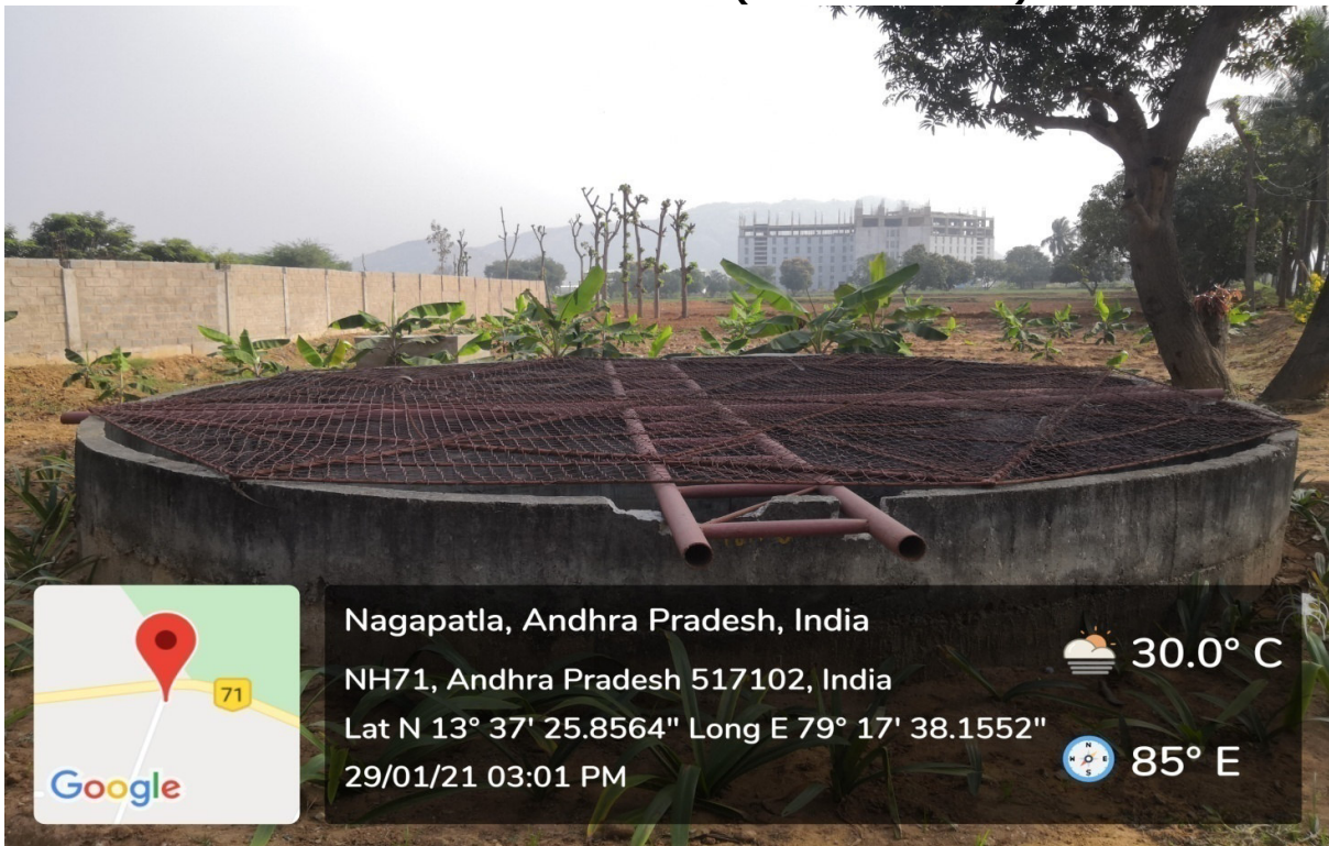
Open Well near the V Block Main Gate (Size: 6.3 m Diameter x 27 m Depth)
