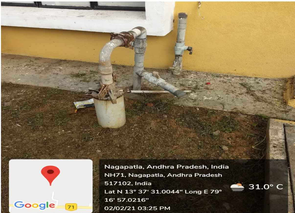
Bore Well-2 at Boys Hostel (6.5" Diameter)
