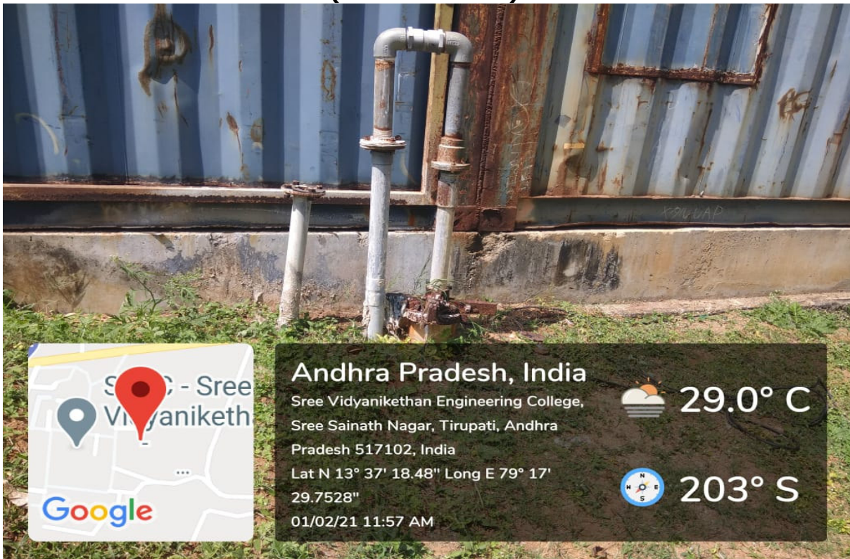
Bore Well near Indoor Stadium (6.5" Diameter)
