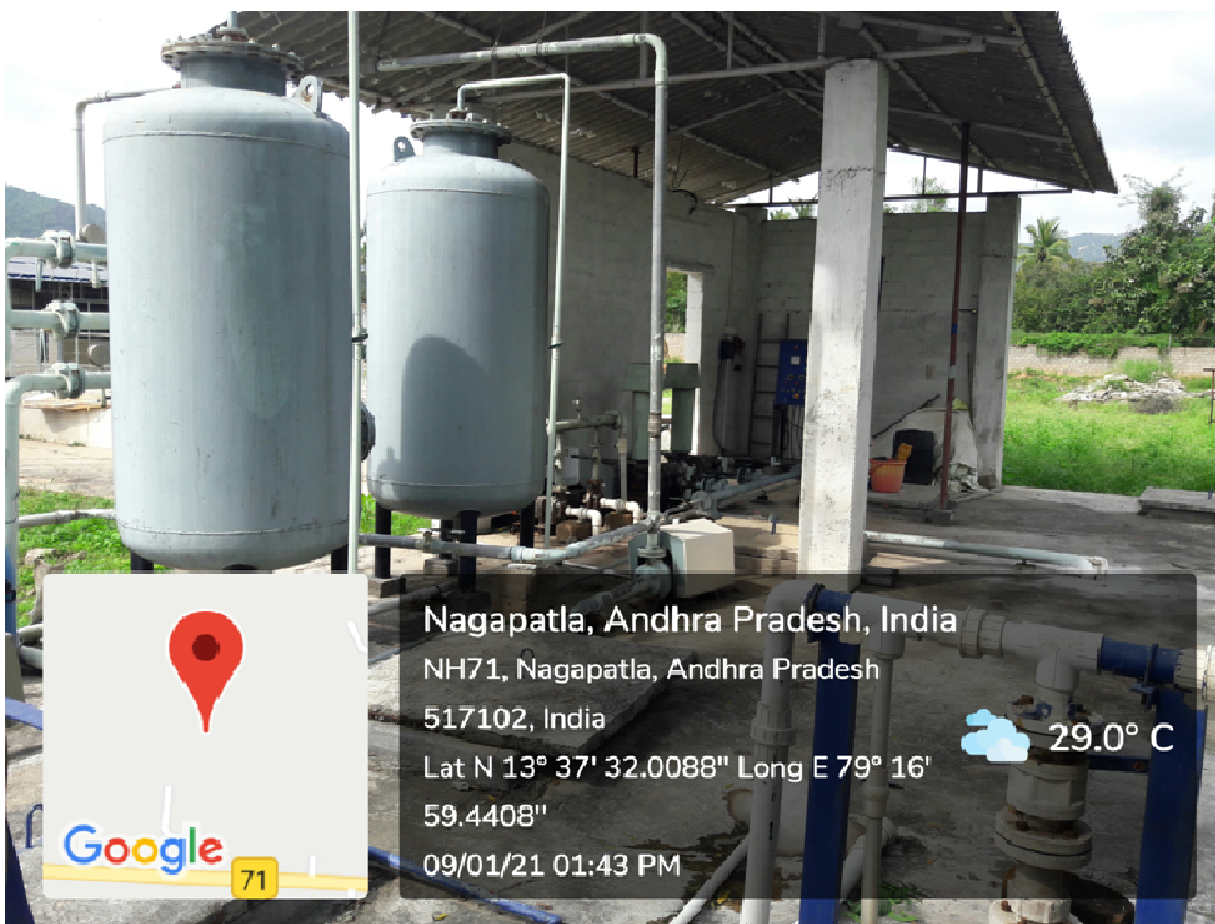
Sewage Treatment Plant of 200 KLD Capacity at Boys Hostels
