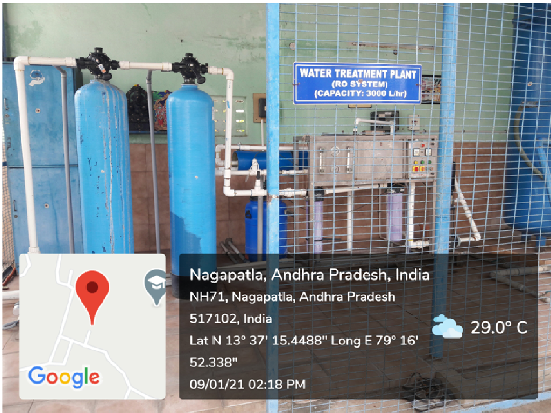
Reverse Osmosis (RO) System (3000 Liters per Hour Capacity) at Girls Hostel Premises
