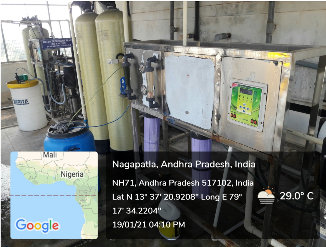
Two Reverse Osmosis (RO) Systems (1000 and 2000 Liters per Hour Capacity) at College Premises
