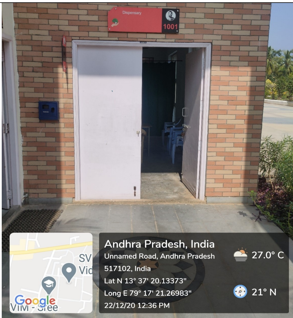
Dispensary Facility (Room No. 1001)
