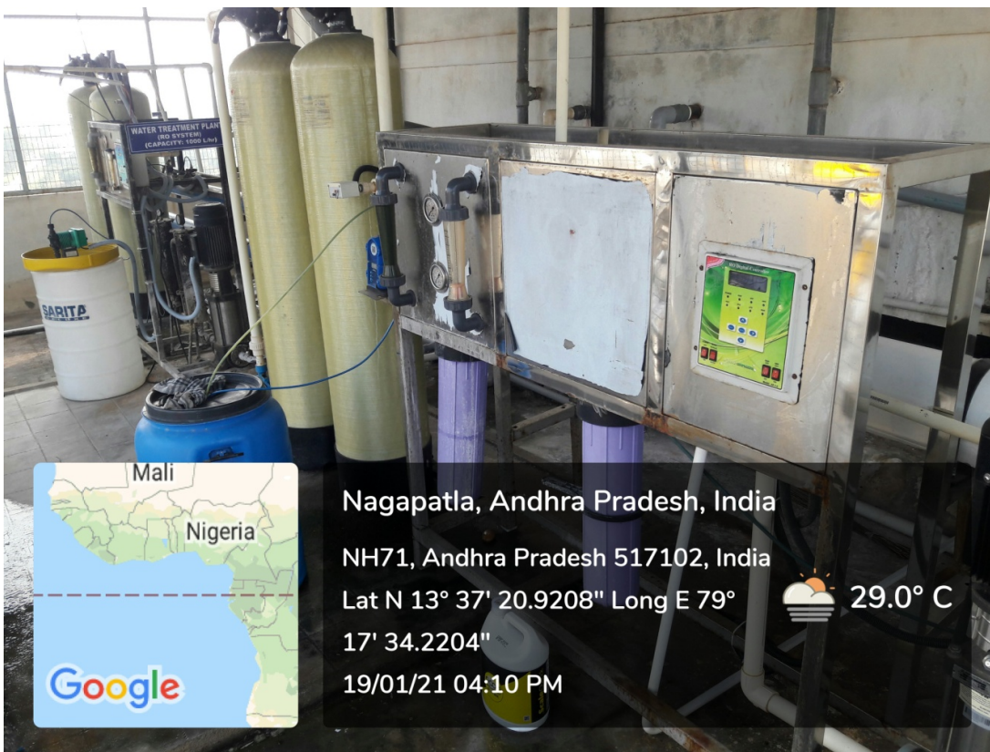
Two Reverse Osmosis (RO) Systems (1000 and 2000 Liters per Hour Capacity) at College Premises
