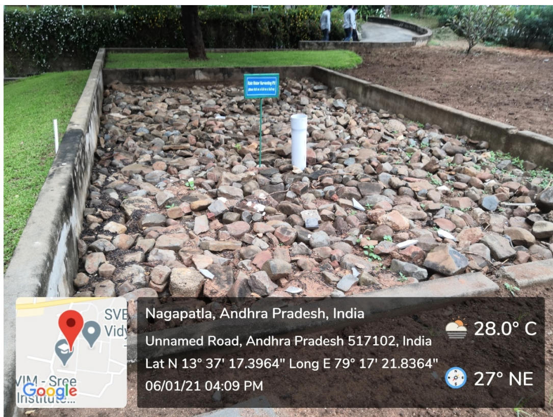
Rainwater Harvesting Pit in front of MNS Block (Size: 9.0 m x 5.0 m x 3.6 m)
