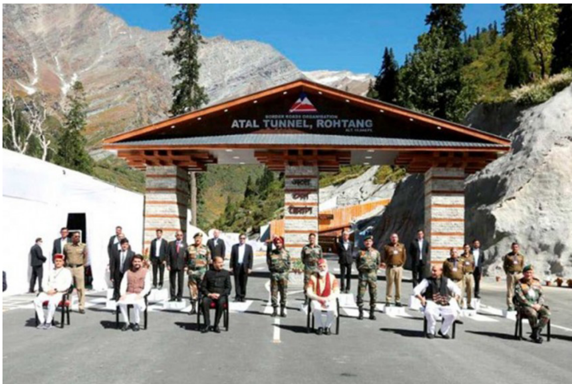
Photographs of World Longest Tunnel – ATAL Tunnel, Rohtang, Himachal Pradesh, India
