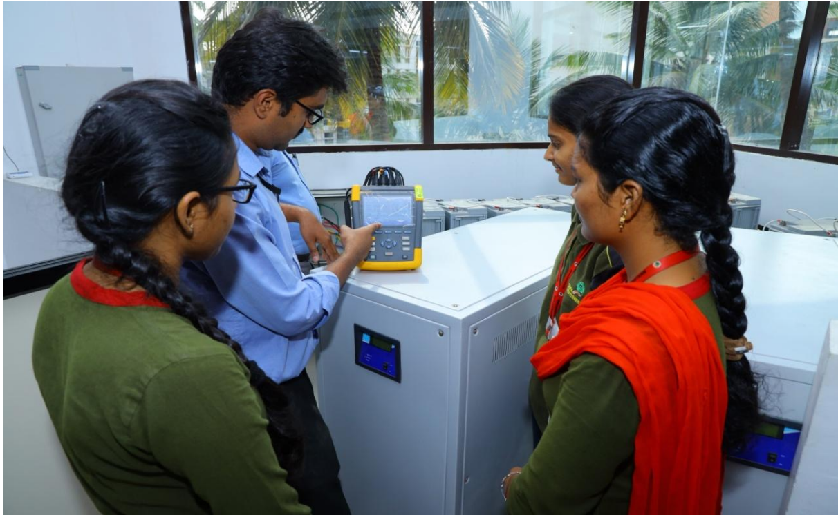
Power quality analysis in Inverters room
