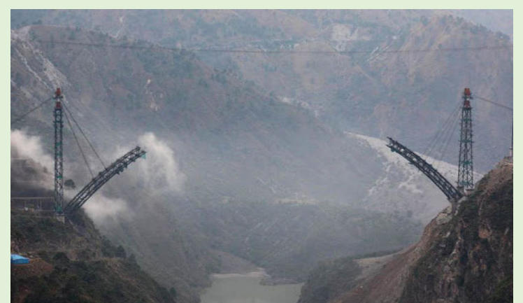
Photograph of World's Highest Railway Bridge - Chenab Railway Bridge Construction as part of presentation
