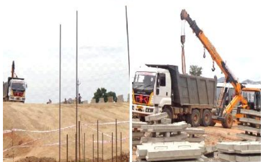
Construction Equipment at the Site
