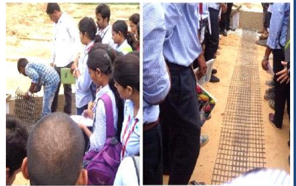
Construction of Geogrid Reinforced Earth
