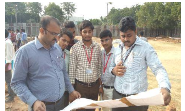
Dr. M. V. Subba Reddy and Mr. D. V. Purushotham explaining the Drawing Details to Students at the Construction Site of Indoor Stadium in SVEC Campus
