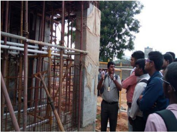
Mr. D. V. Purushotham explains the Shuttering and Scaffolding at the Construction Site of Sri Shirdi Sai Baba Temple besides SVEC Campus
