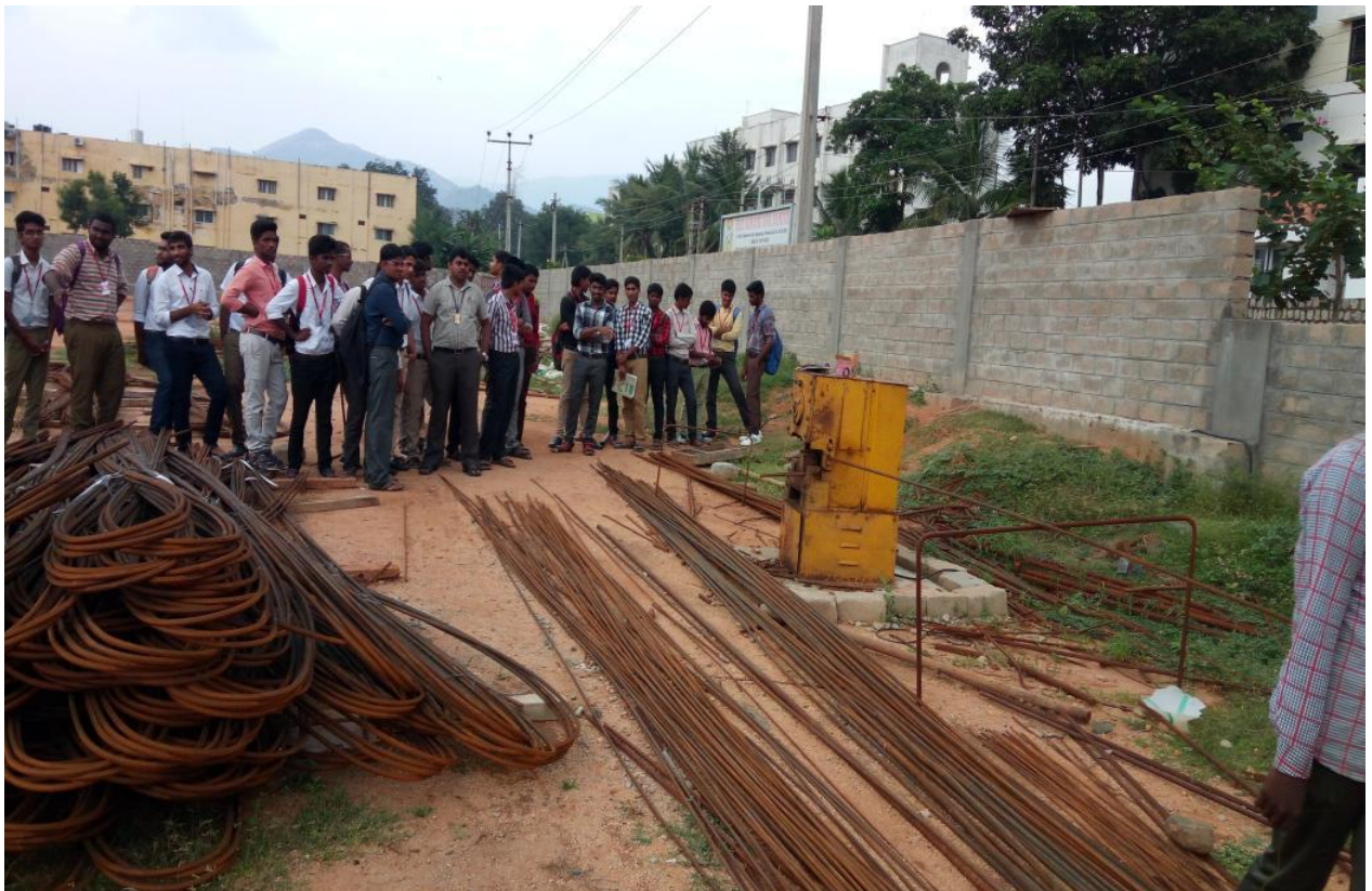
Mr. D. V. Purushotham showing the Use of Bar Cutting Machine at the Construction Site of Sri Shirdi Sai Baba Temple besides SVEC Campus
