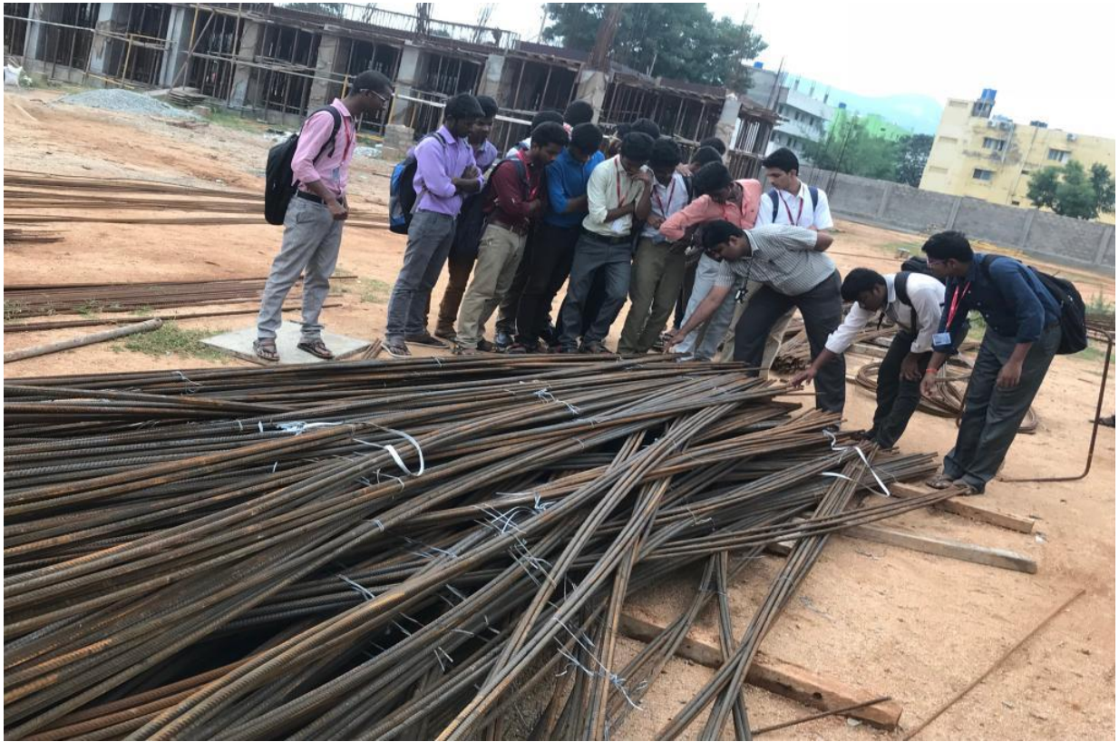
Mr. D. V. Purushotham explains the Usage of HYSD Steel Reinforcement at the Construction Site of Sri Shirdi Sai Baba Temple besides SVEC Campus
