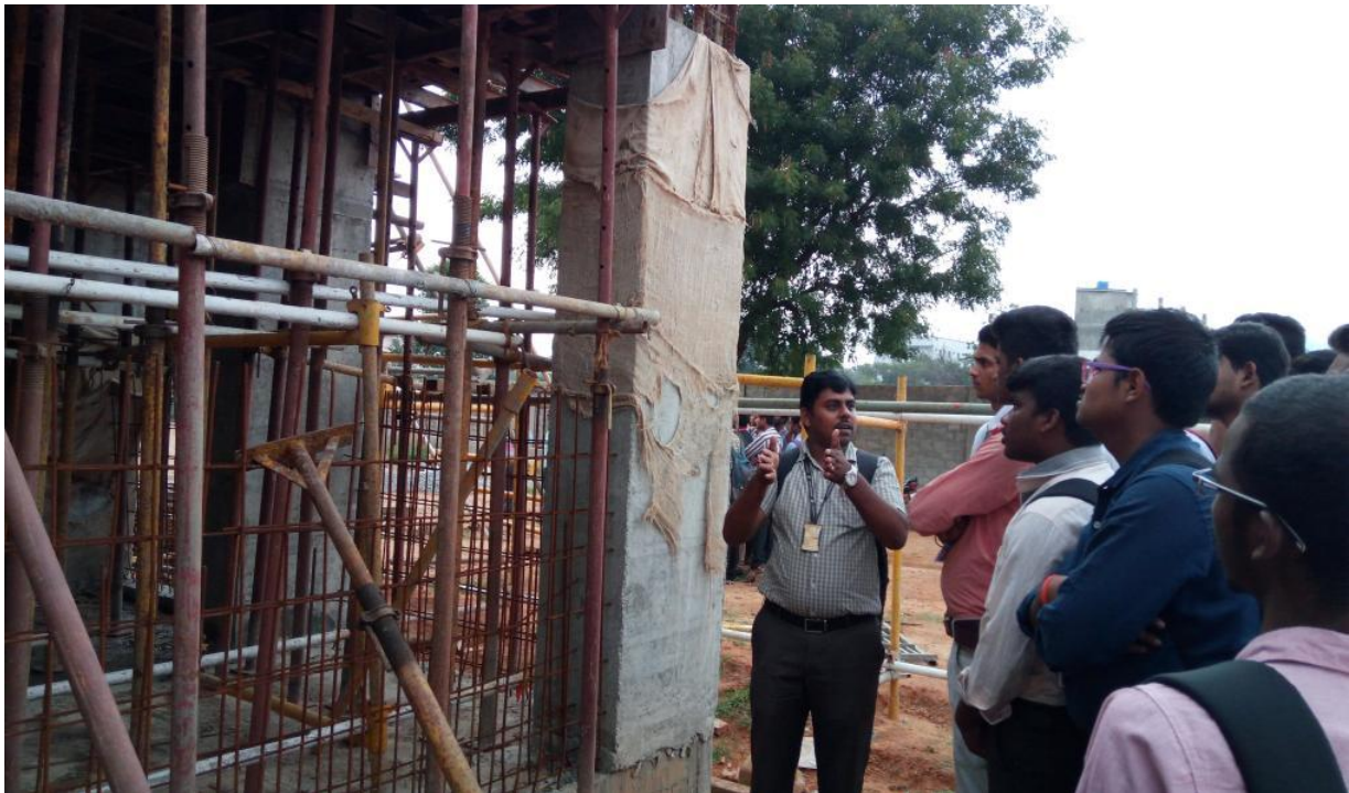
Mr. D. V. Purushotham explains the Shuttering and Scaffolding at the Construction Site of Sri Shirdi Sai Baba Temple besides SVEC Campus
