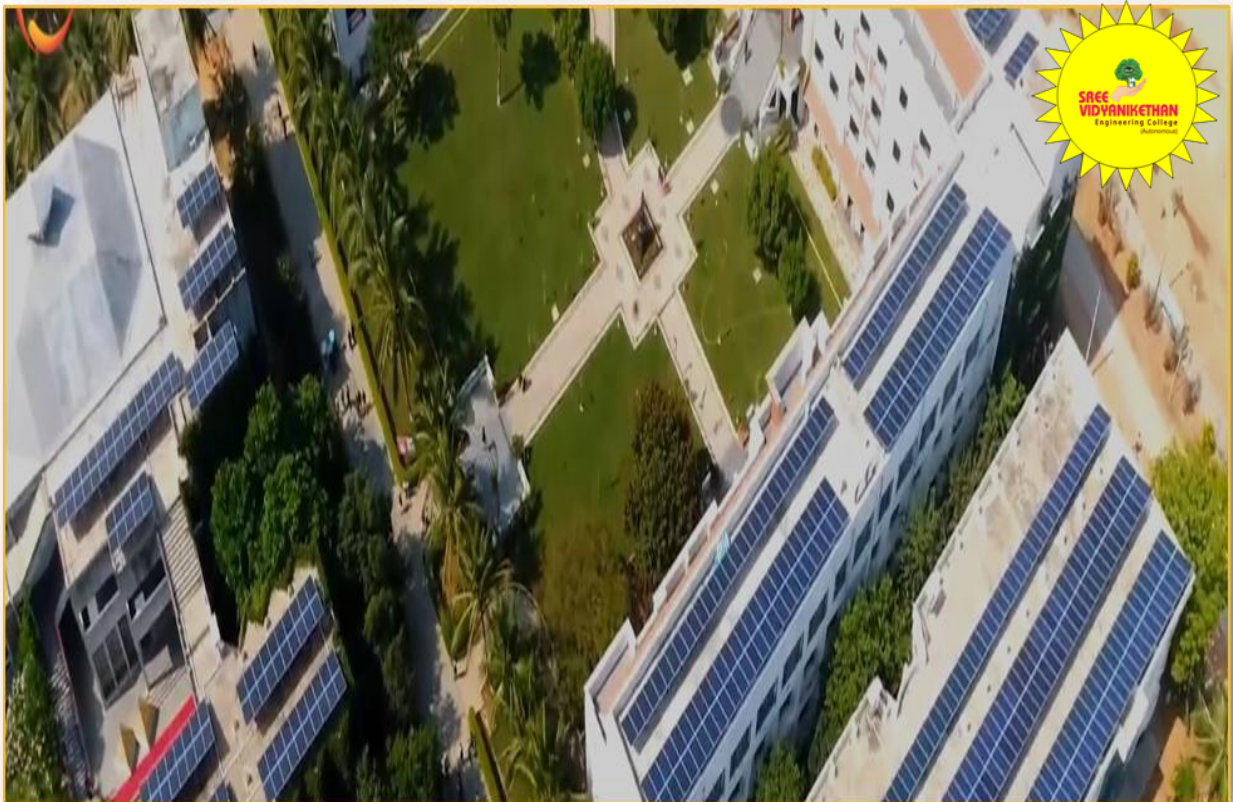
Arial view of Roof Top Solar PV System, Sree Vidyanikethan Engineering College
