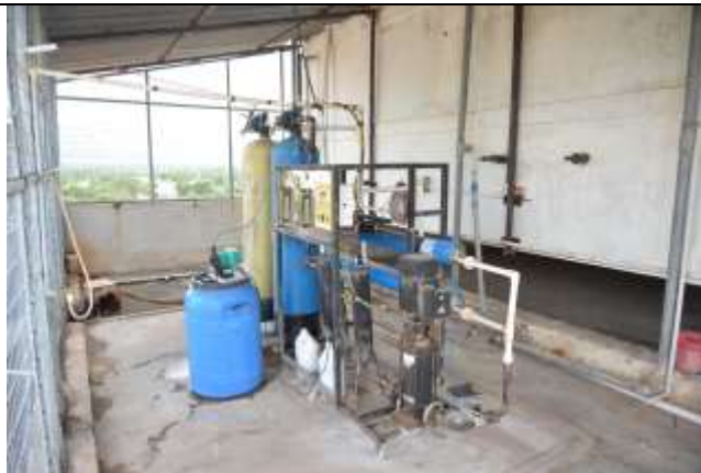
Reverse Osmosis (RO) System (1000 Liters per hour capacity) at College
