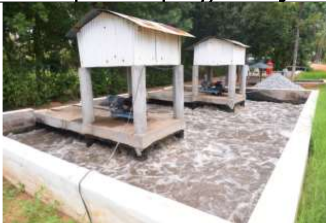
Sewage Treatment Plant of 150 KLD Capacity
