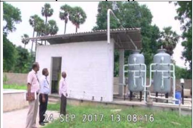
Sewage Treatment Plant of 200 KLD Capacity
