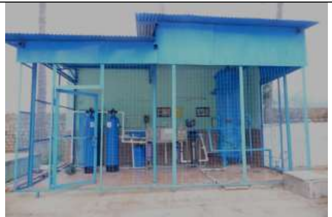
Reverse Osmosis (RO) System (1000 Liters per hour capacity) at Hostel
