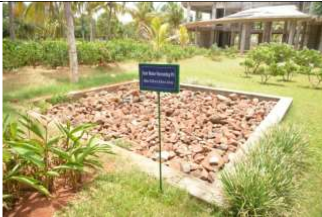
Rainwater Harvesting Pit at New Canteen (Size: 5.25 m x 5.0 m x 3.6 m)
