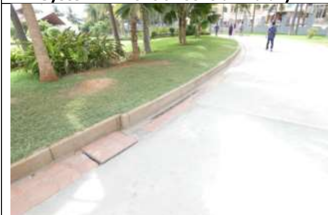
Rain Water Collection and Conveyance System on the Way to Canteen
