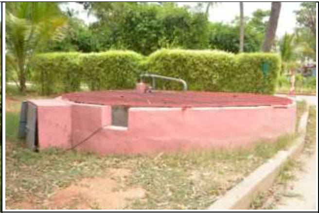
Open Well near Main Gate (Size: 4.3 m Diameter x 20 m Depth) with Bore (4" Diameter)
