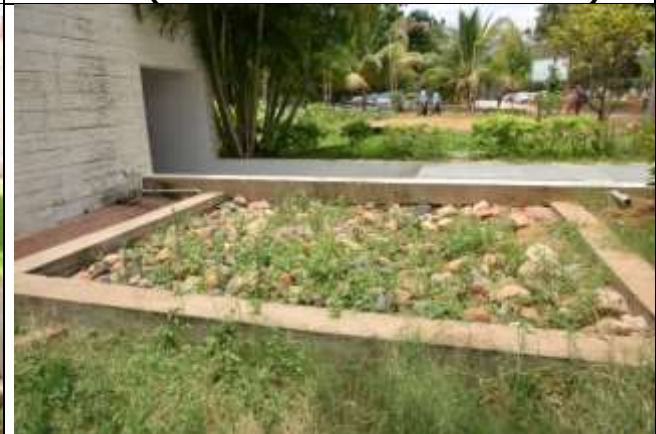
Rainwater Harvesting Pit at PAT Office (Size: 4.0 m x 4.0 m x 3.6 m)
