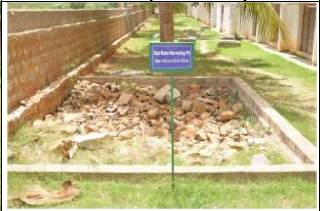
Rainwater Harvesting Pit beside MNS Block (Size: 5.25 m x 5.0 m x 3.6 m)
