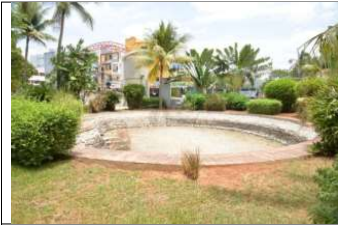
Rain Water Harvesting Pond at Main Gate (Size: 14.5 m Diameter X 1.5 m Depth)
