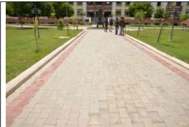
Porous/Permeable Concrete Paver Tiles Separated by Joints at MNS Block to Infiltrate Rainwater
