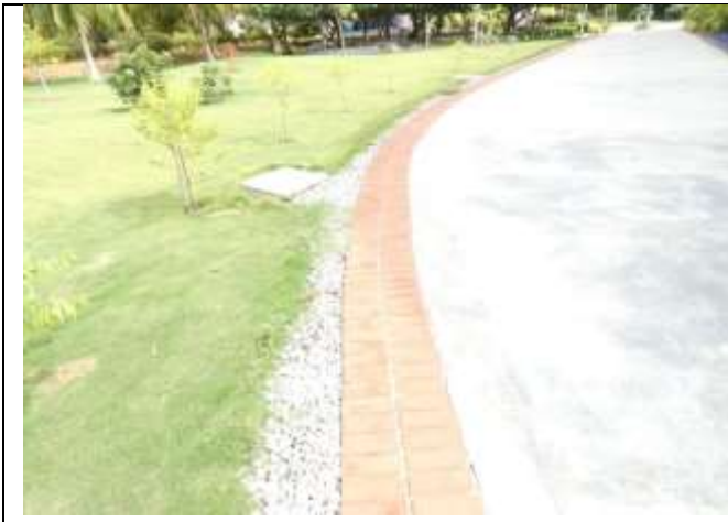
Rain Water Collection and Conveyance System at Central Library
