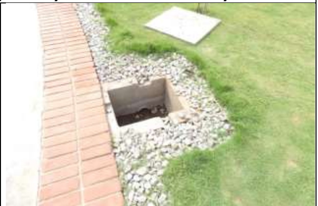
Rain Water Collection Point at Central Library
