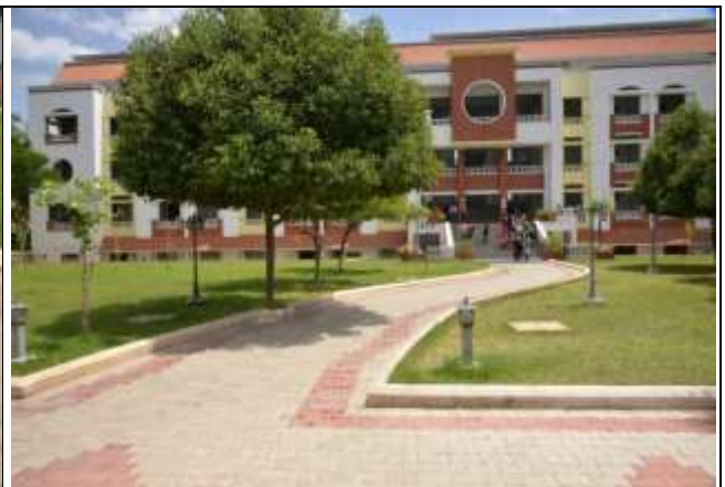
Porous/Permeable Concrete Paver Tiles Separated by Joints at MNS Block to Infiltrate Rainwater
