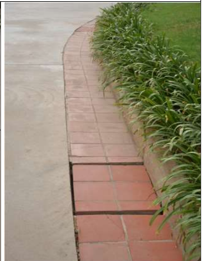
Rain Water Collection and Conveyance System Opposite to M-Block
