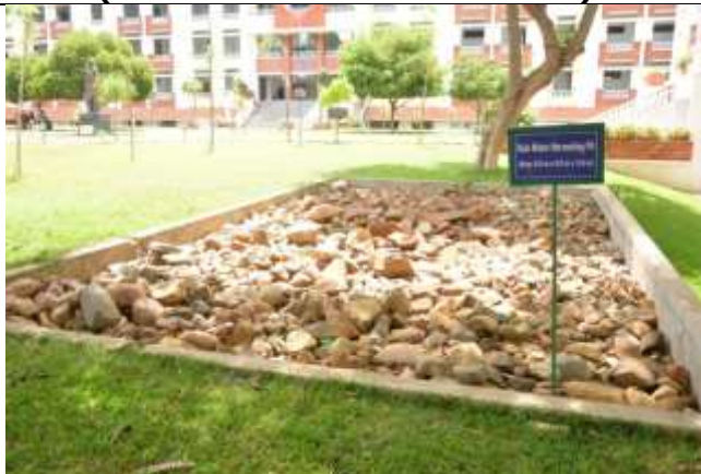
Rainwater Harvesting Pit at MNS Block (Size: 9.0 m x 5.0 m x 3.6 m)
