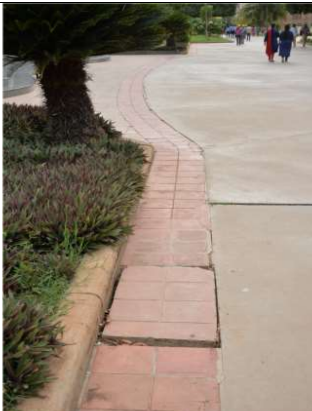
Rain Water Collection and Conveyance System in Front of M-Block
