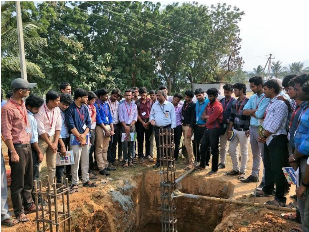
A Field Visit to Construction Sites of Indoor Stadium and Hostel Building at Sree Vidyanikethan Engineering College Campus
