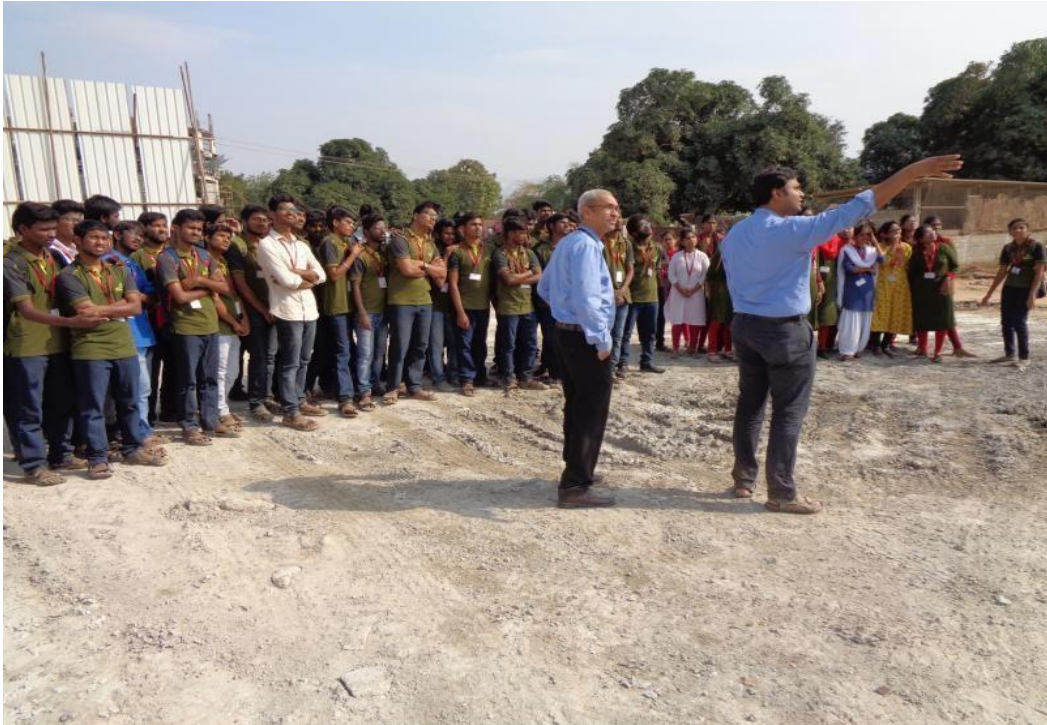
A Field Visit to the Construction Site of College Hostel Building at Sree Vidyanikethan Engineering College Campus
