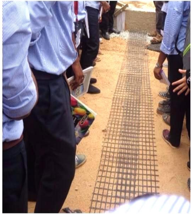
Construction of Geogrid Reinforced Earth
