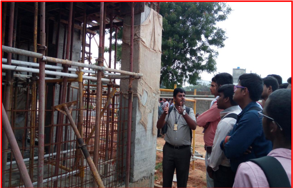
Mr. D. V. Purushotham explaining the Shuttering and Scaffolding at the Construction Site of Sri Shirdi Sai Baba Temple
