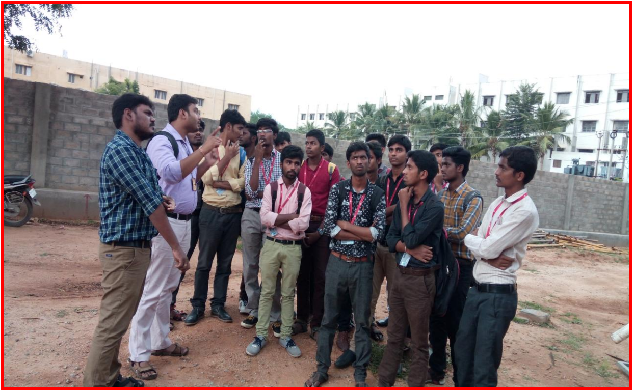
Mr. M. Gokulnath and Mr.V. Prem Kumar explaining the Construction Details at the Construction Site of Sri Shirdi Sai Baba Temple
