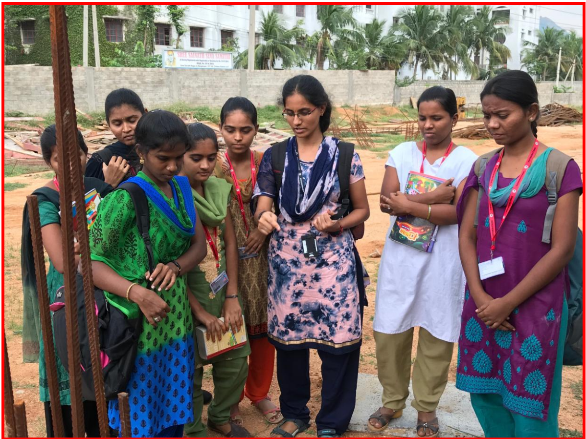
Ms. P. Ramya explains the Construction Procedure of RCC Isolated Footings at the Construction Site of Sri Shirdi Sai Baba Temple
