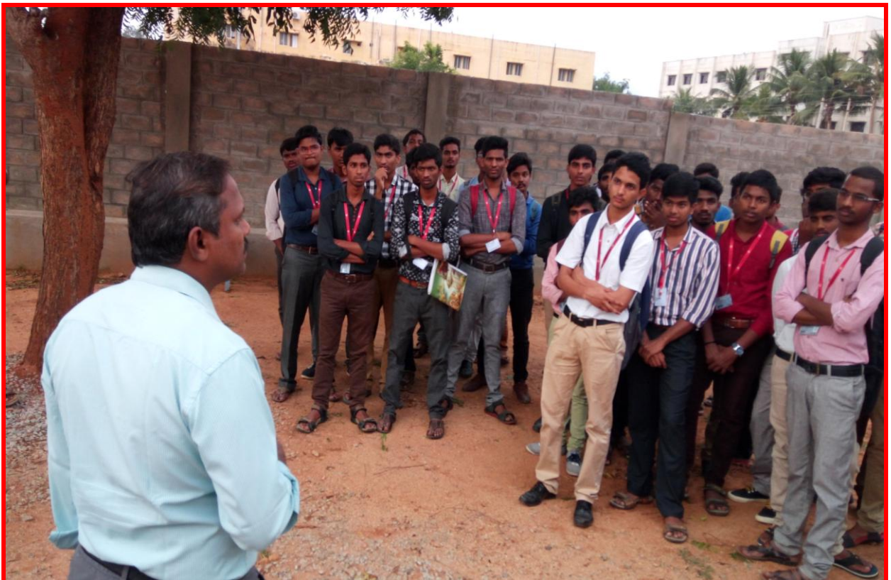
Dr. O. Eswara Reddy explaining the Importance of Shear Wall Design in the Construction Site of Sri Shirdi Sai Baba Temple
