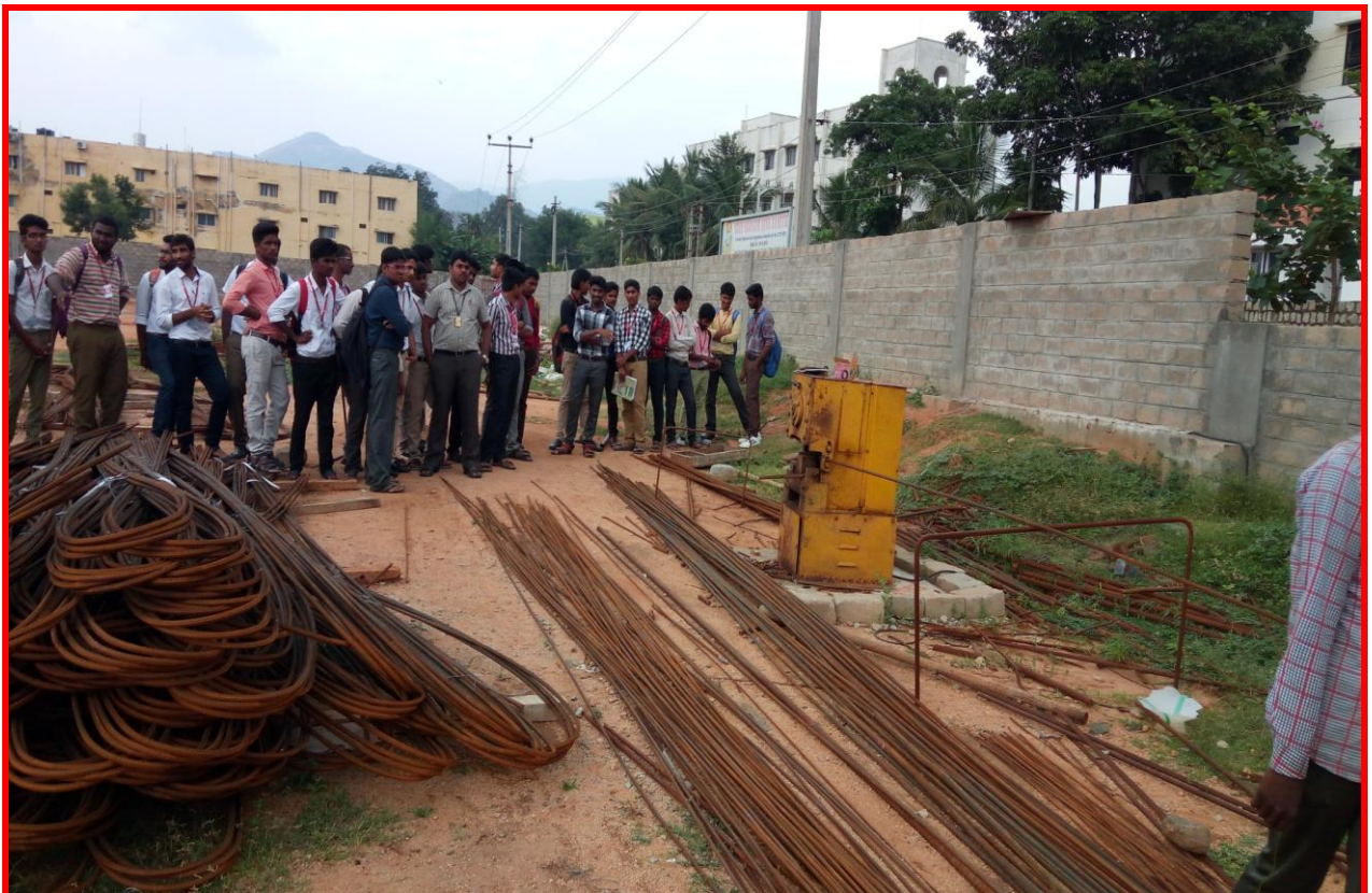
Mr. D. V. Purushotham showing the Use of Bar Cutting Machine at the Construction Site of Sri Shirdi Sai Baba Temple
