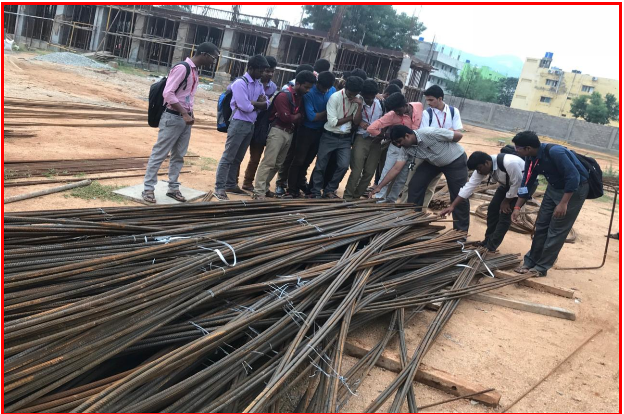
Mr. D. V. Purushotham explaining the Usage of HYSD Steel Reinforcement at the Construction Site of Sri Shirdi Sai Baba Temple
